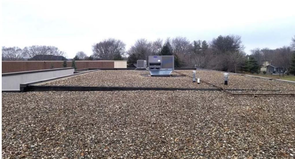
CENTER - LOOKING WEST
