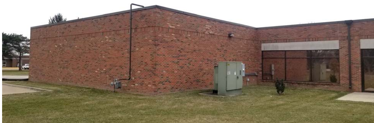
NORTHWEST CORNER - EAST SIDE
