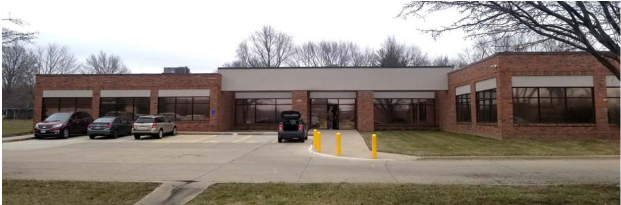
SOUTH - BUILDING FRONT ENTRANCE
