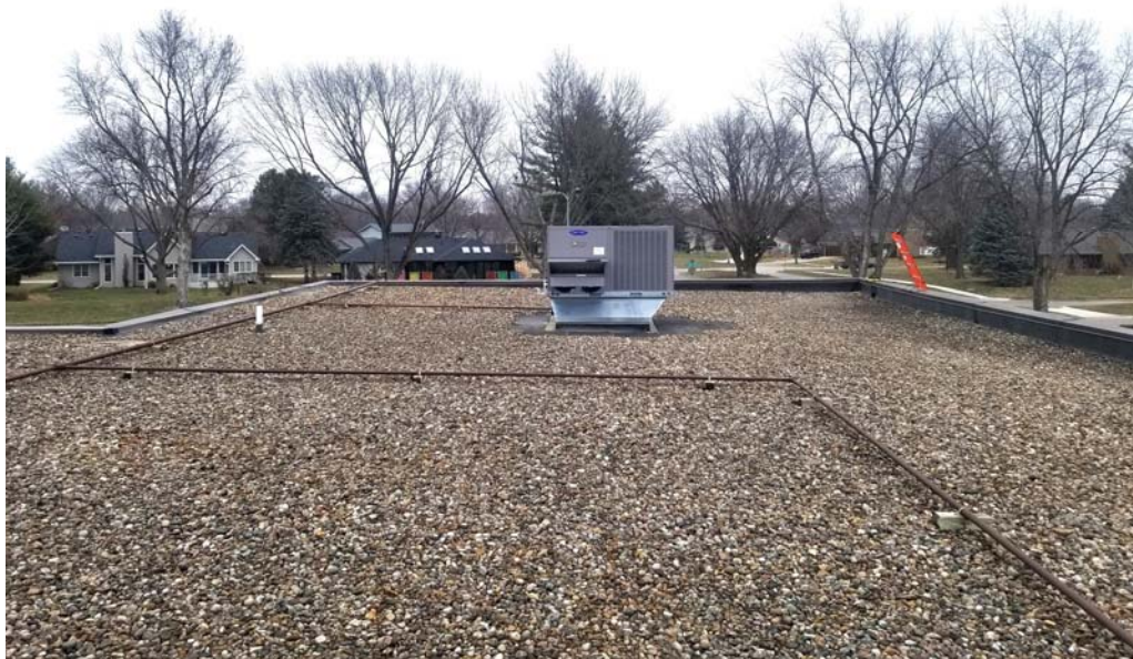
EAST WING - LOOKING NORTH
