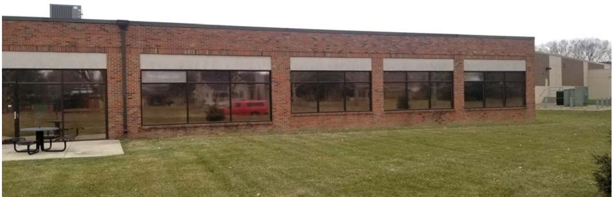
NORTH CORNER - WEST SIDE
