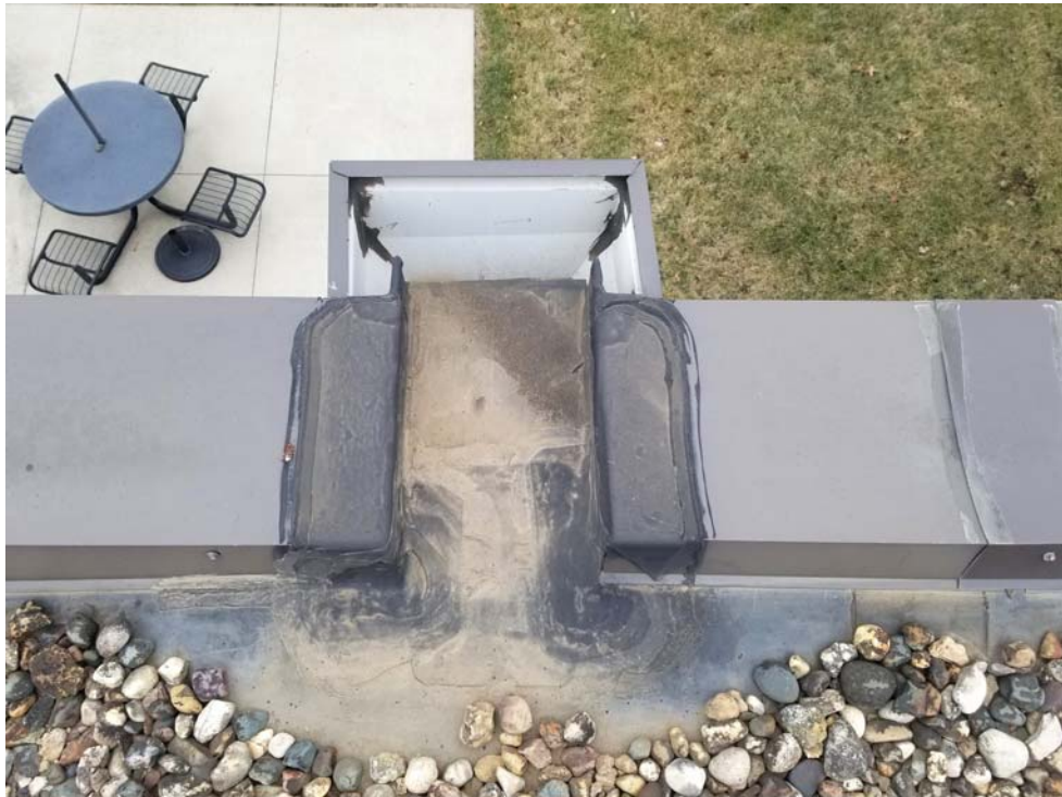
OPEN TOP SCUPPERS AT NORTH CENTER
