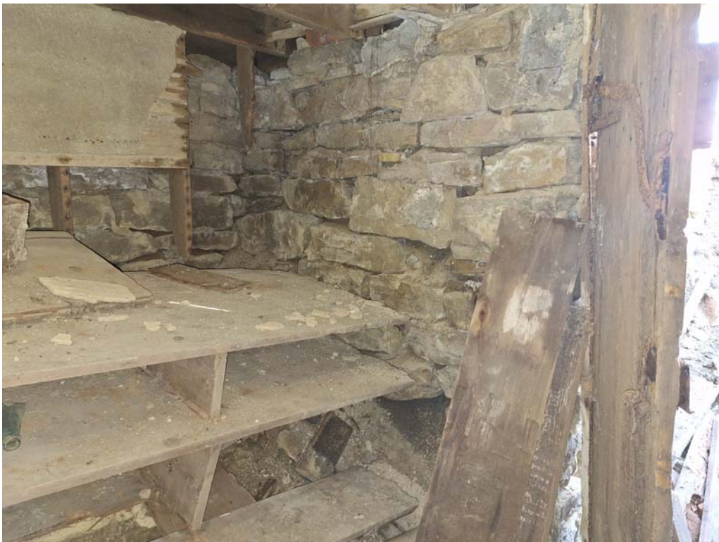
STONE FOUNDATION NEEDING UNDERPIN & INFILL - LEFT SIDE OF BSMT DOOR
