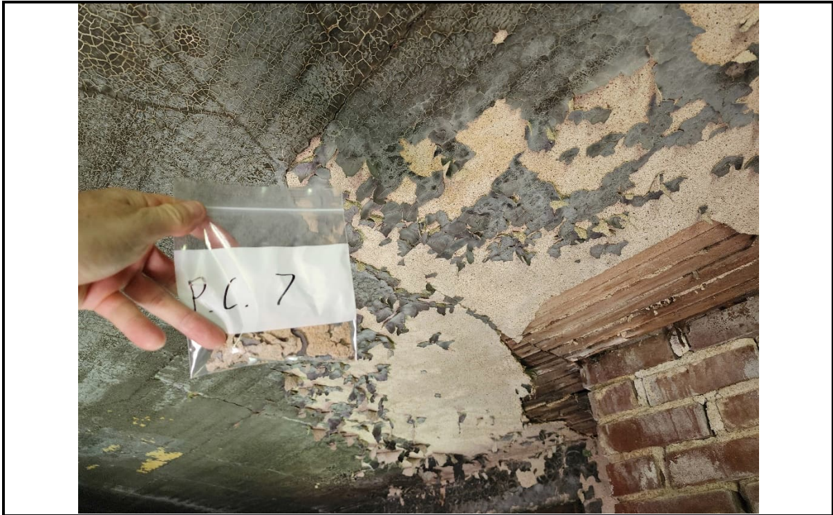
Photo 13: PC 7: Confirmed lead-containing green paint on the plaster kitchen ceiling.
