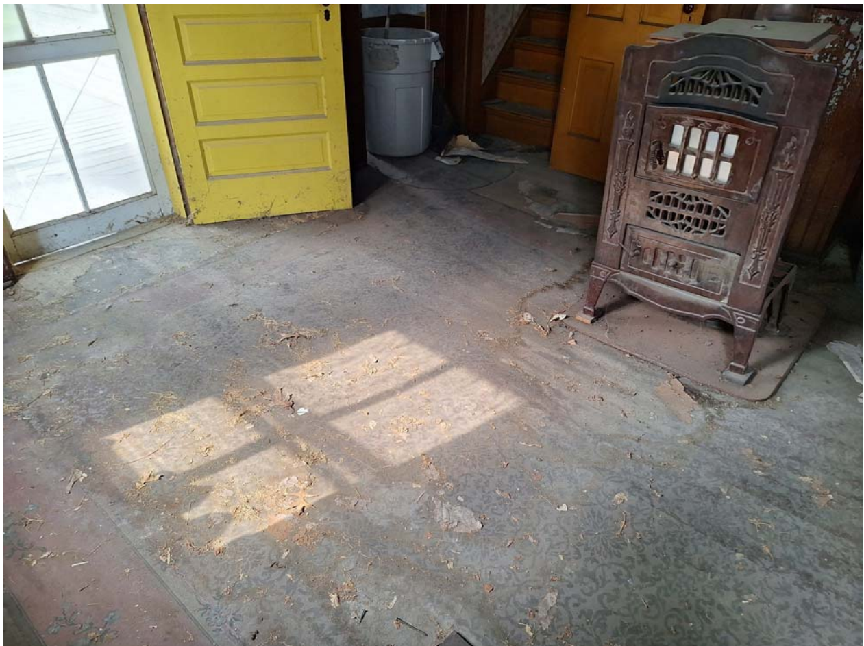
ENTRANCE ROOM SAGGING ROTTED FLOOR TO BE REPLACED
