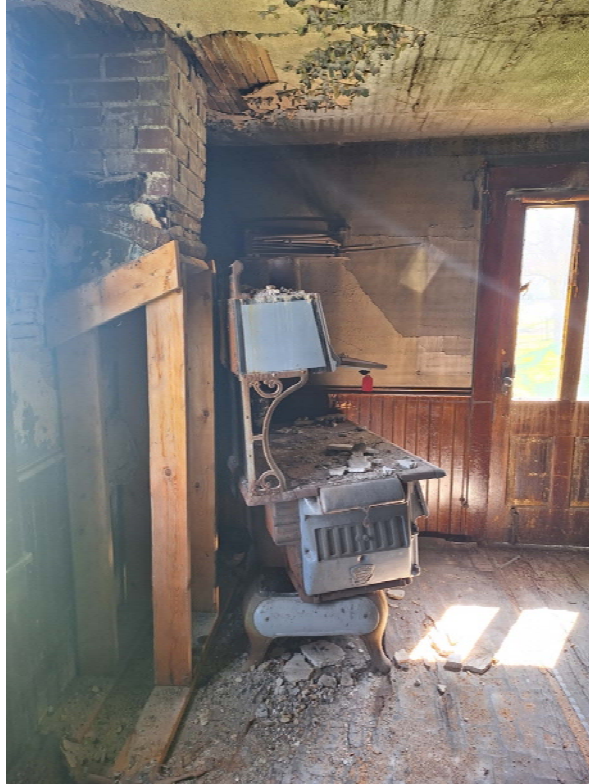
NORTH KITCHEN CHIMNEY AND PLASTER TO BE REPAIRED
