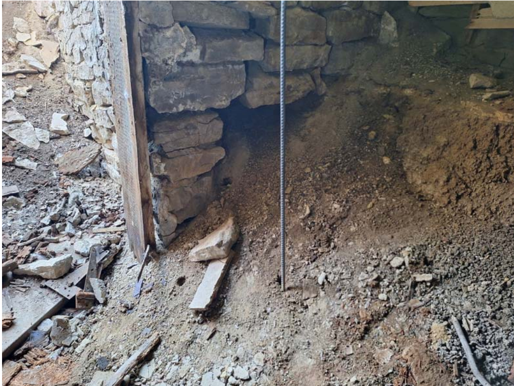
STONE FOUNDATION NEEDING UNDERPIN & INFILL - RIGHT SIDE OF BSMT DOOR
