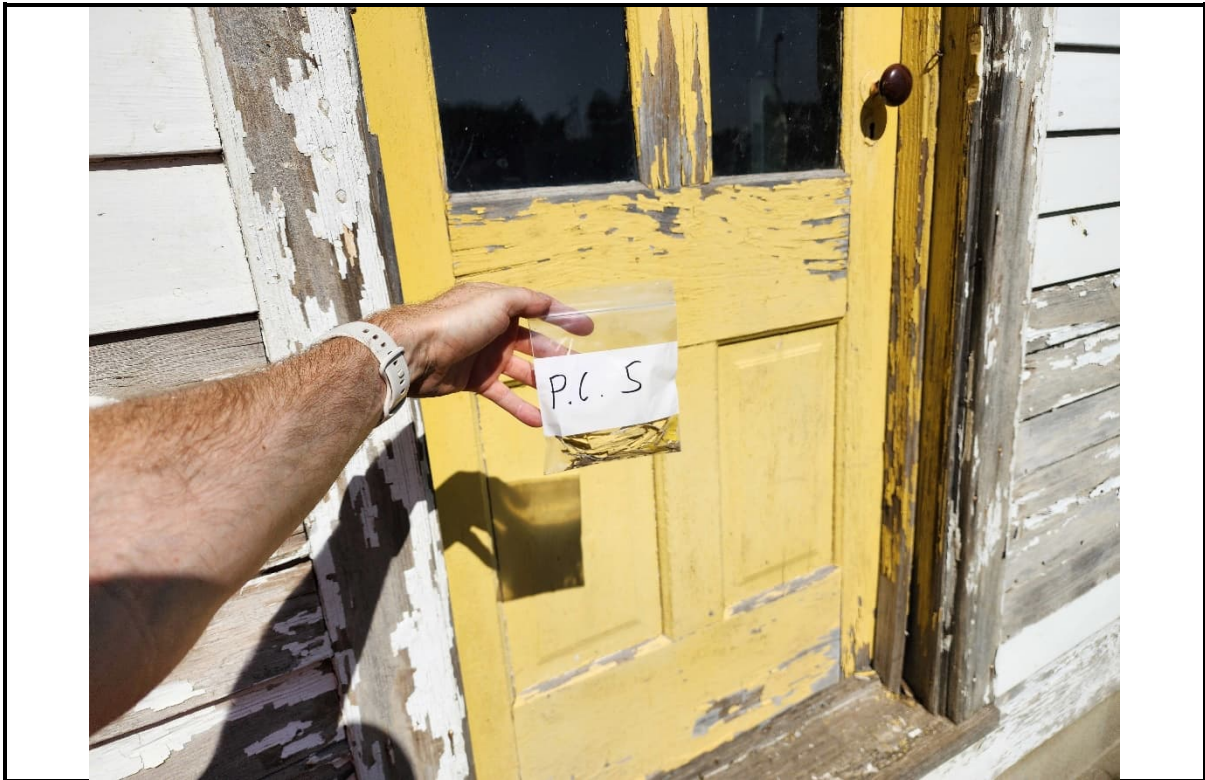
Photo 11: PC 5: Confirmed lead-containing yellow paint on the front and side door of the house.
