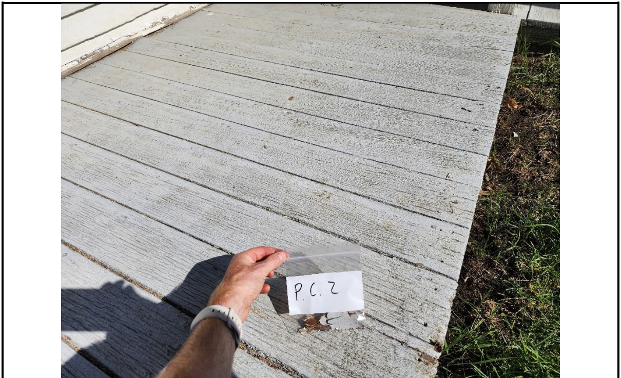
Photo 8: PC 2: Confirmed lead-containing blue paint on the front porch floor.
