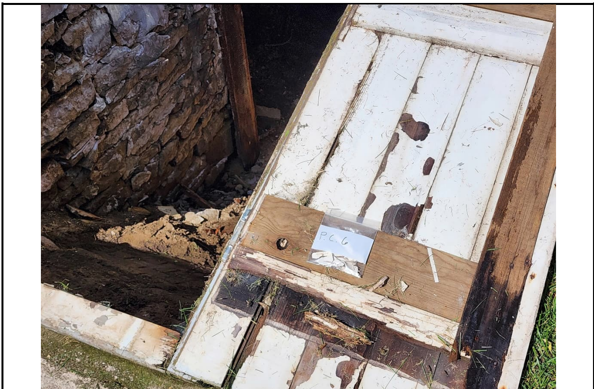
Photo 12: PC 6: Confirmed lead-containing white paint on the wood basement cellar door.
