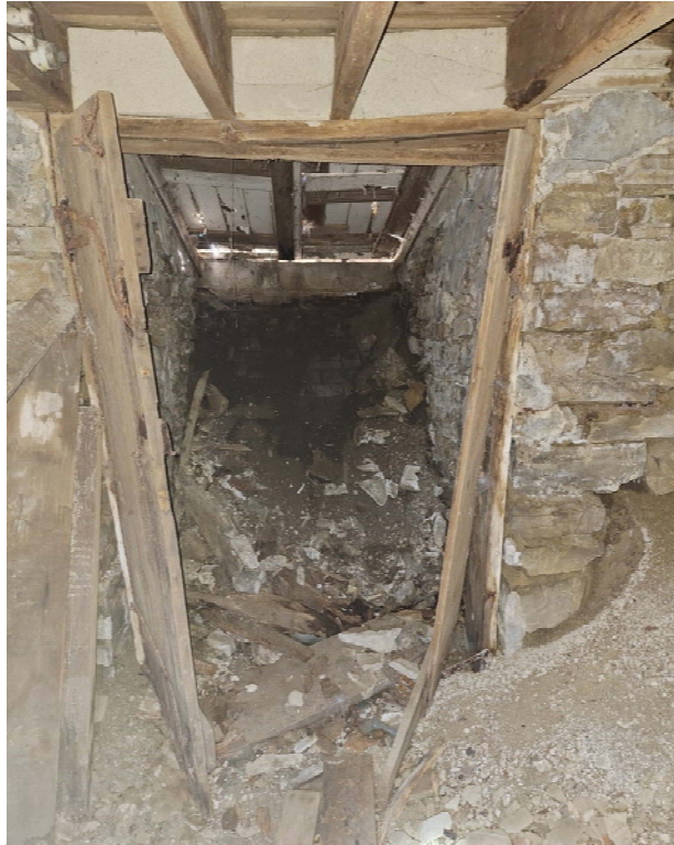
BASEMENT CELLARWAY - EXTERIOR STAIRS & SAGGING SILL BEAM
