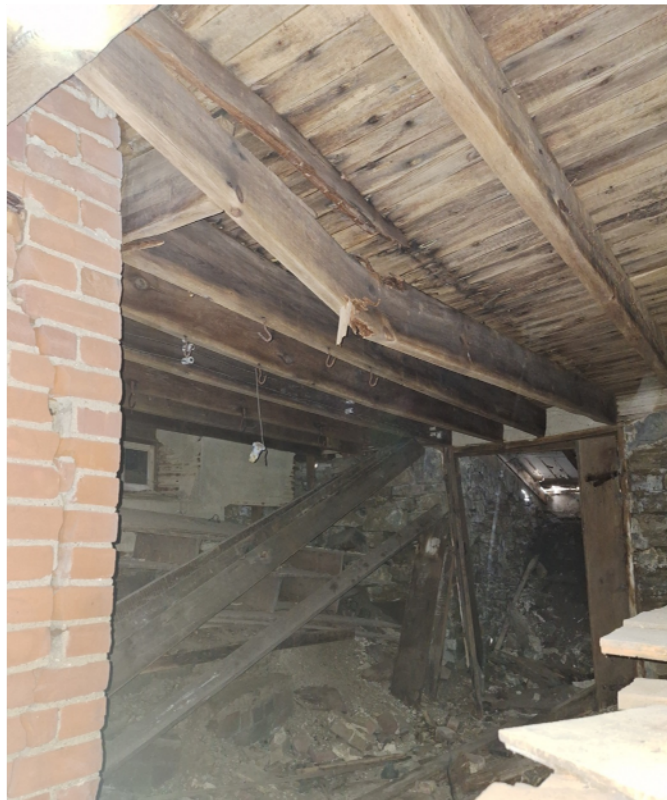
ROTTED FLOOR JOISTS AND FLOORING
