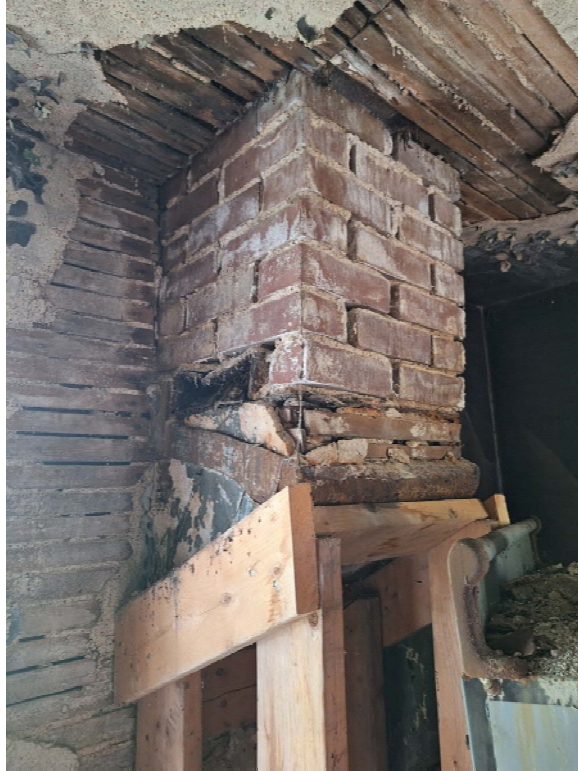
NORTH KITCHEN CHIMNEY TO BE REPAIRED
