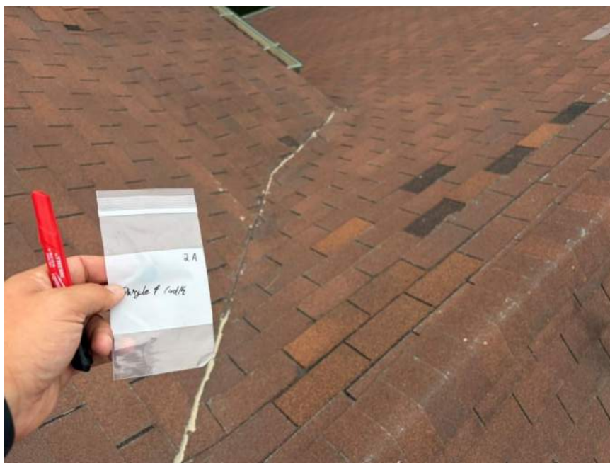
2A-Shingle, Middle Upper Roof SW Facing Side-None Detected
