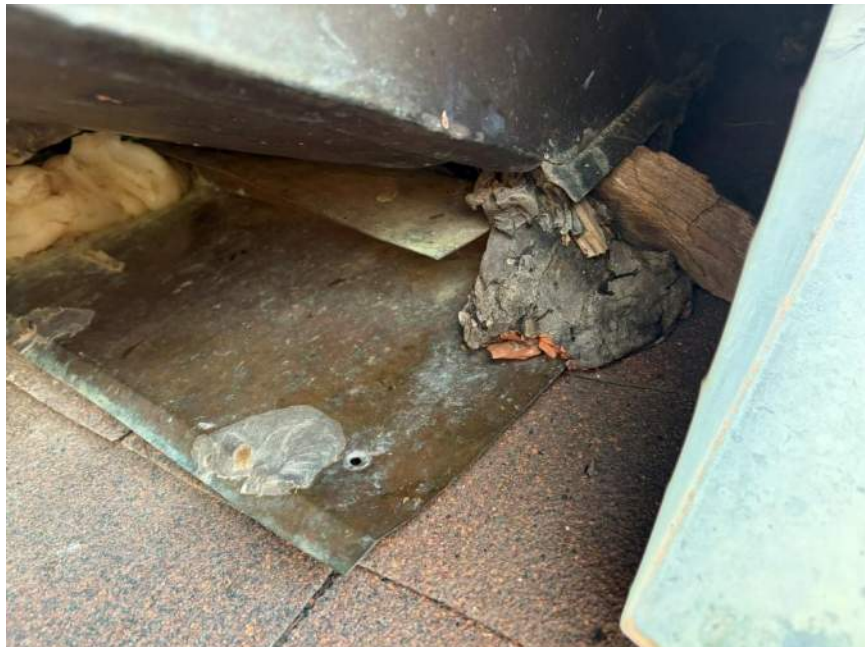
9A-Roofing Tar, Middle Upper Roof Southern Overhang-Chrysotile 5%
