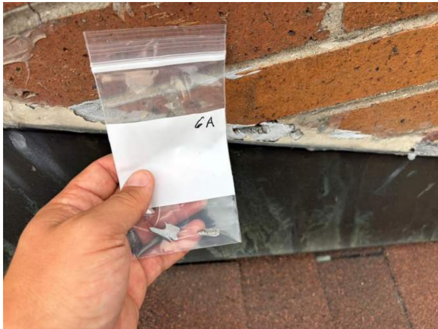
6A-Caulking, Middle Upper Roof NW Side-None Detected
