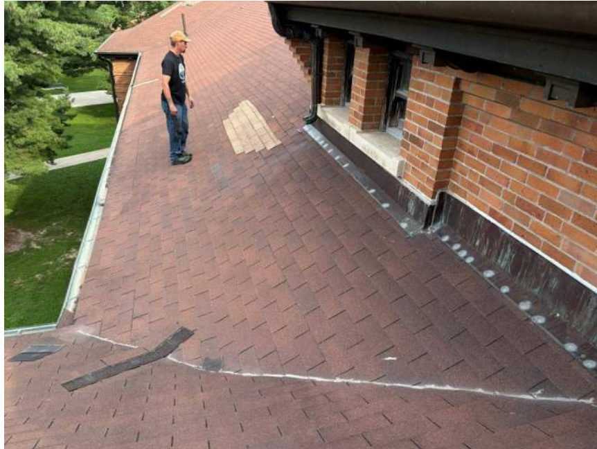
10A-Shingle, North Western, Lower Roof Patch-None Detected
