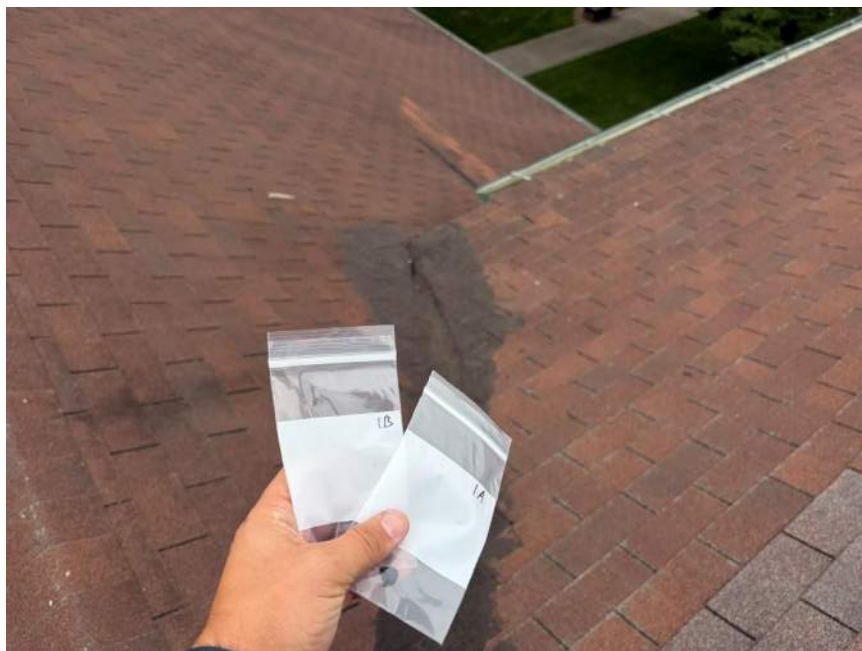
1A-Hard Rubberized Coating, Roof Valley SW Side-None Detected 1B-Hard Rubberized Coating, Roof Valley SW Side-None Detected
