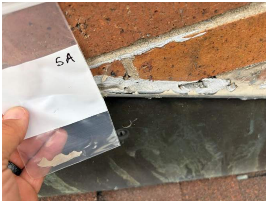
5A-Caulking, Middle Upper Roof NW Facing Side-None Detected
