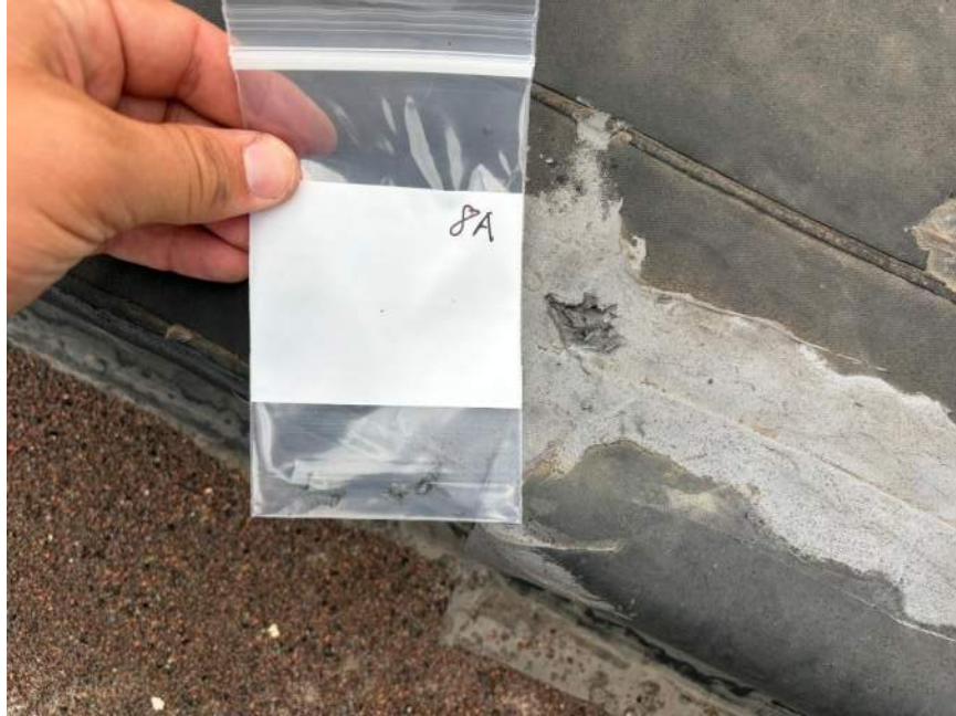
8A-Parapet Tar, Southern Most Flat Roof-None Detected
