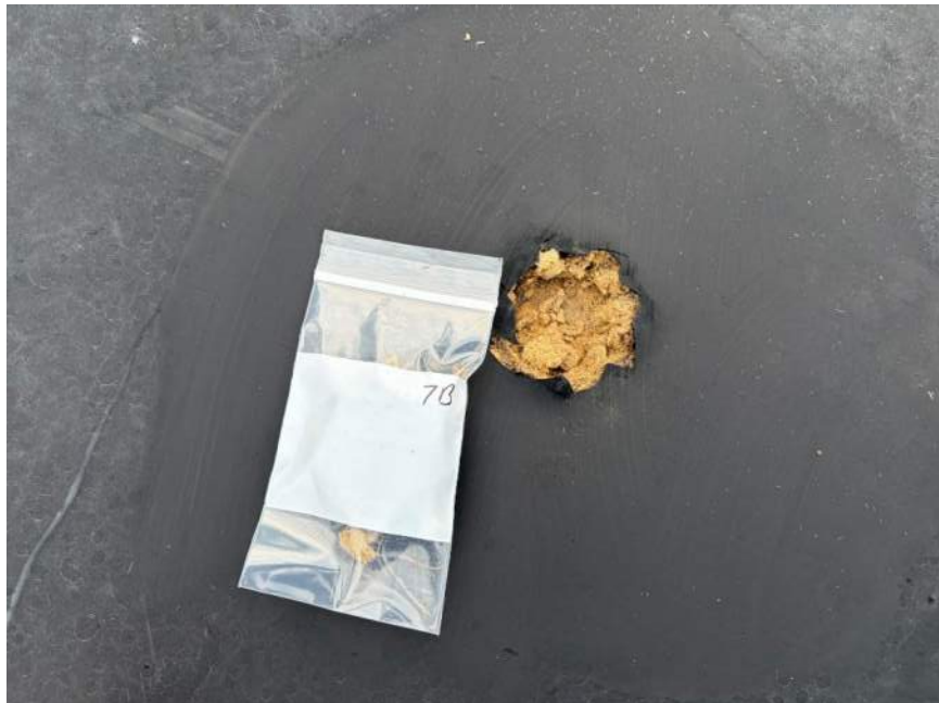
7B-Flat Roofing Core, Southern Most Flat Roof-None Detected
