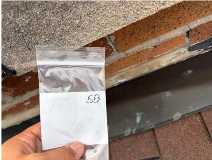
5B-Caulking, Middle Upper Roof NW Facing Side-None Detected
