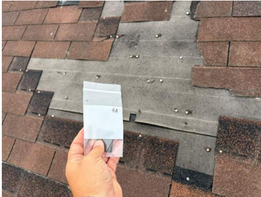
4A-Roofing Felt, Middle Upper Roof NE Facing Side-None Detected
