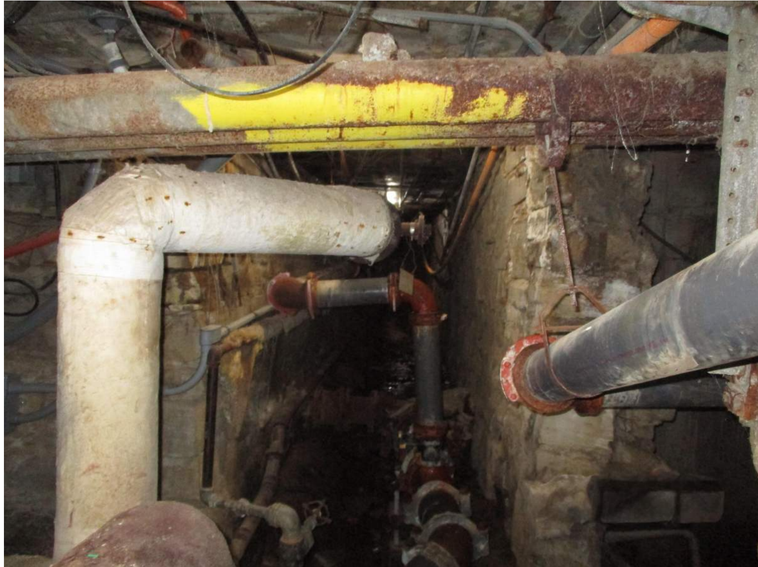
2 PHOTO OF TUNNEL AT SALLYPORT
