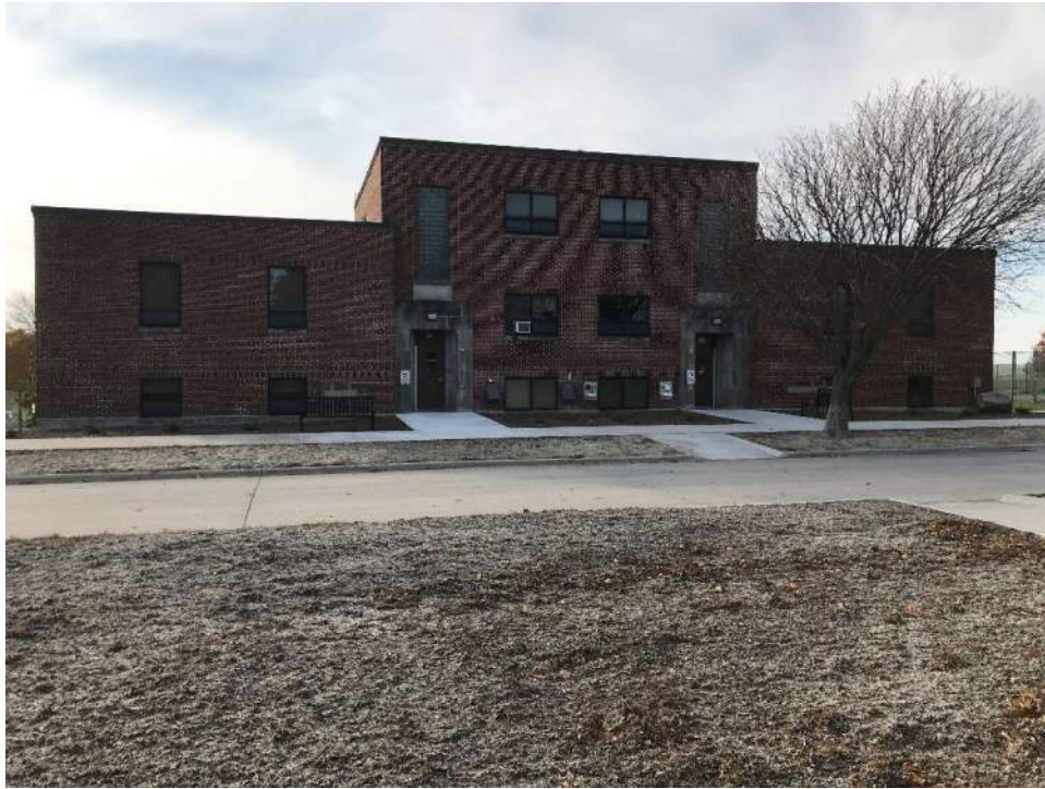
View of Cottages 5 and 6 from the east.
