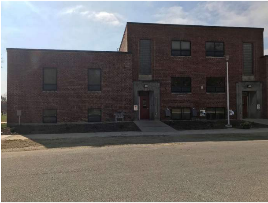
View of Cottage 7 from the east.
