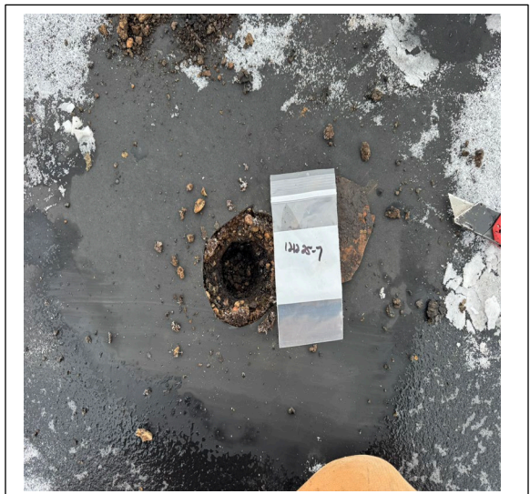
Sample 121225-7: Rubber/adhesive on North end of main roof negative for asbestos.
