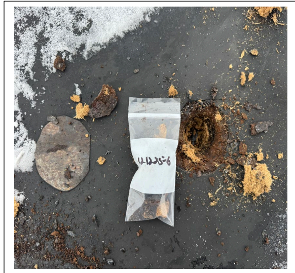
Sample 121225-6: Field on main roof negative for asbestos.
