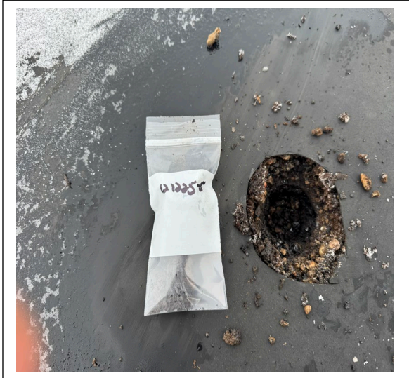
Sample 121225-5: Field on main roof negative for asbestos.
