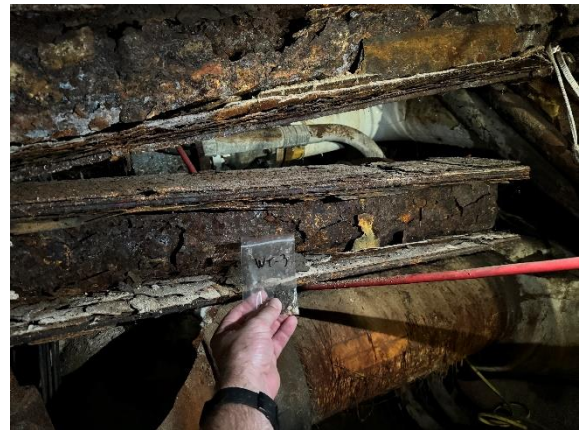
Photo #4 View of the I-Beam Laminations sampled (Non-asbestos).
