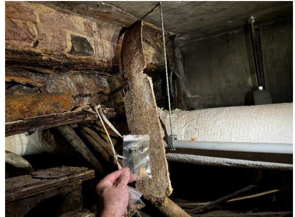
Photo #2 View of the Expansion Joint Fiberboard sampled (Non-asbestos).
