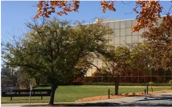
Photo #1 View of the Wallace Building.
