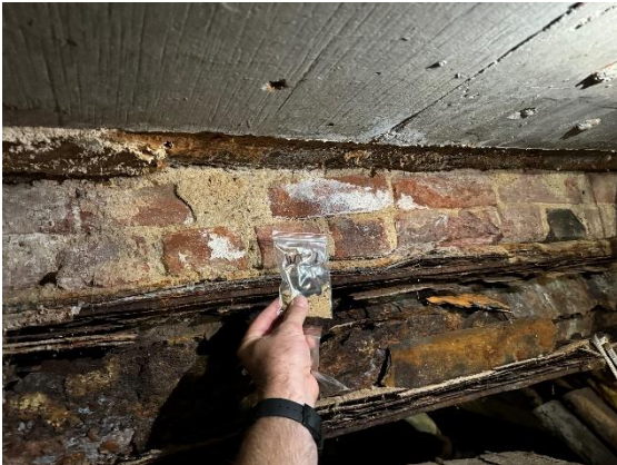
Photo #3 View of the Brick Mortar "Header" sampled (Non-asbestos).
