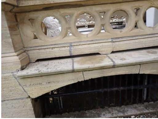
21, 22. Views of cast iron ventilation guard
