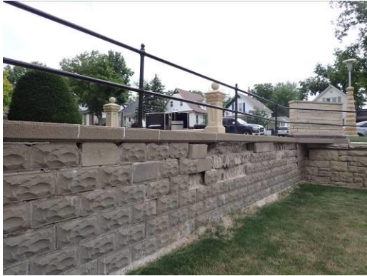
39, 40. Failing retaining walls
