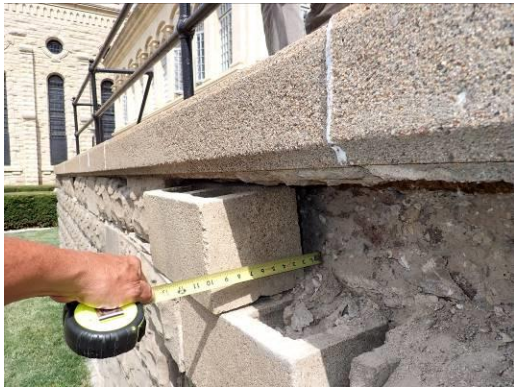
41, 42. Close up of wall failure
