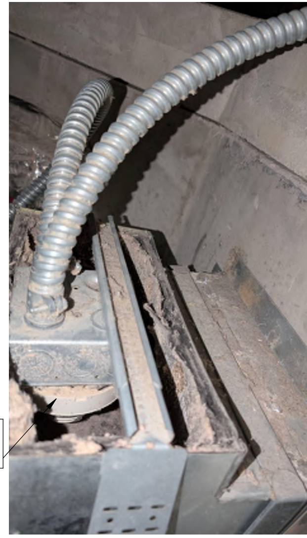
EXISTING SMOKE DETECTOR INSTALLED AT END OF DUCT. REPLACE DETECTOR WITH NEW.
