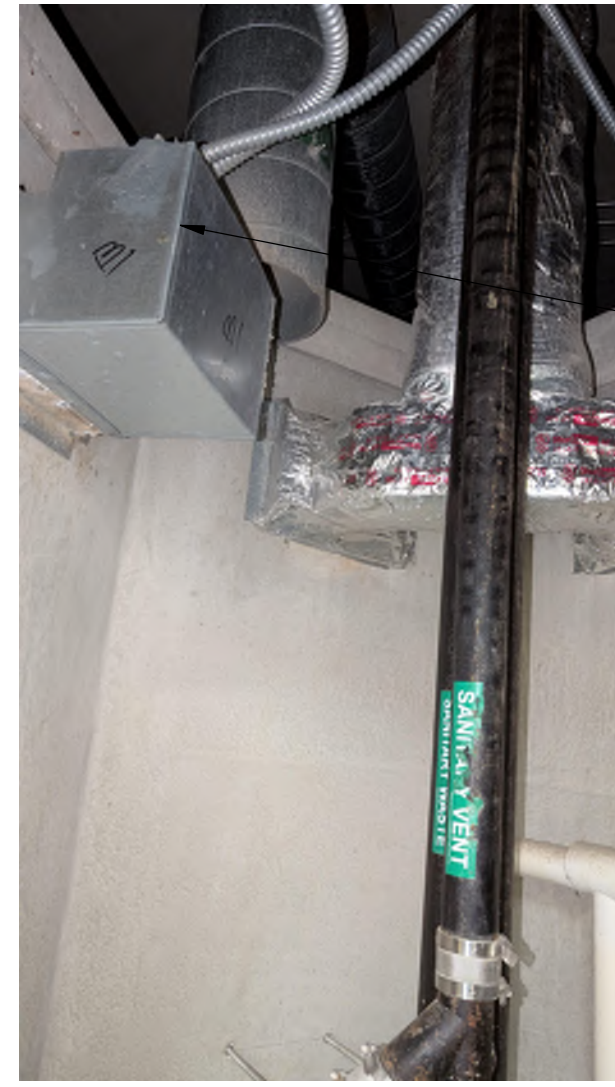
EXISTING DETECTOR INSTALLED AT TOP OF DUCT.
