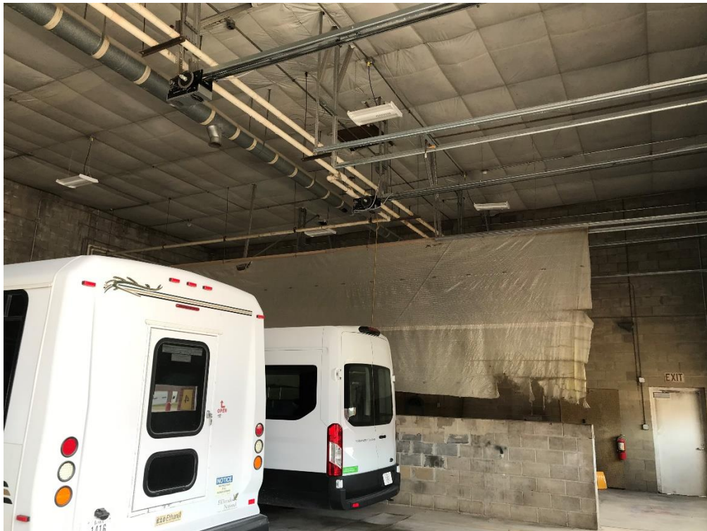
View of interior of the Dispatch Garage.
