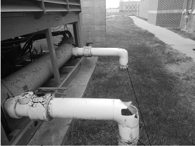
EXISTING CONCRETE PAD
