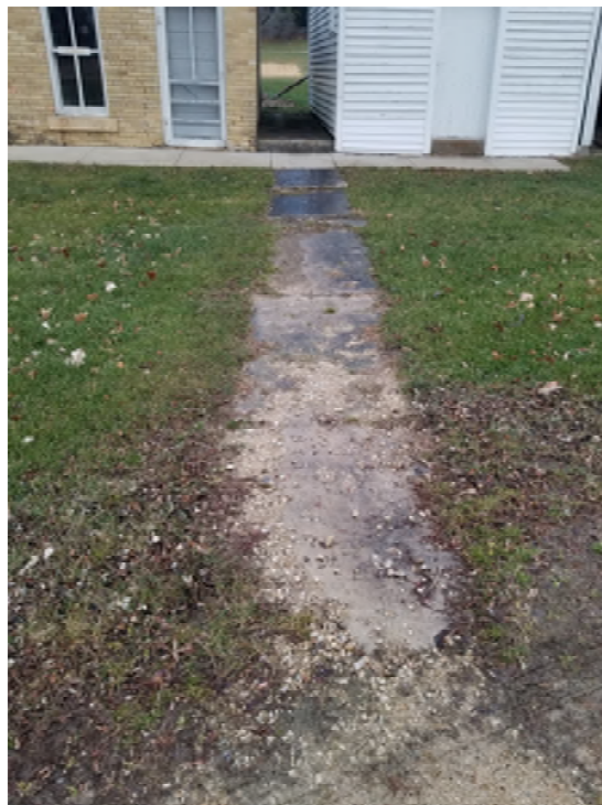
NORTH PAVERS -WEST RUN
