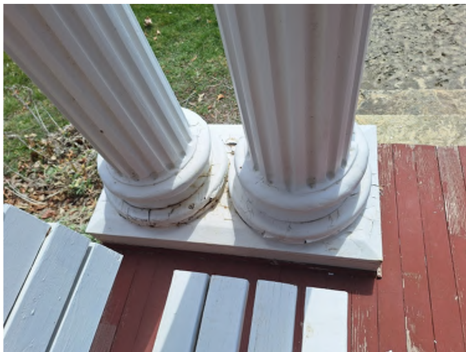
EAST COLUMN BASES - BACK SIDE
