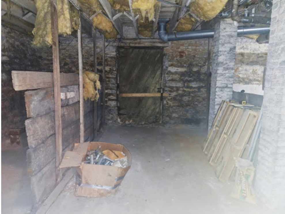
EAST BASMENT ROOM - EXTERIOR CELLARWAY DOOR
