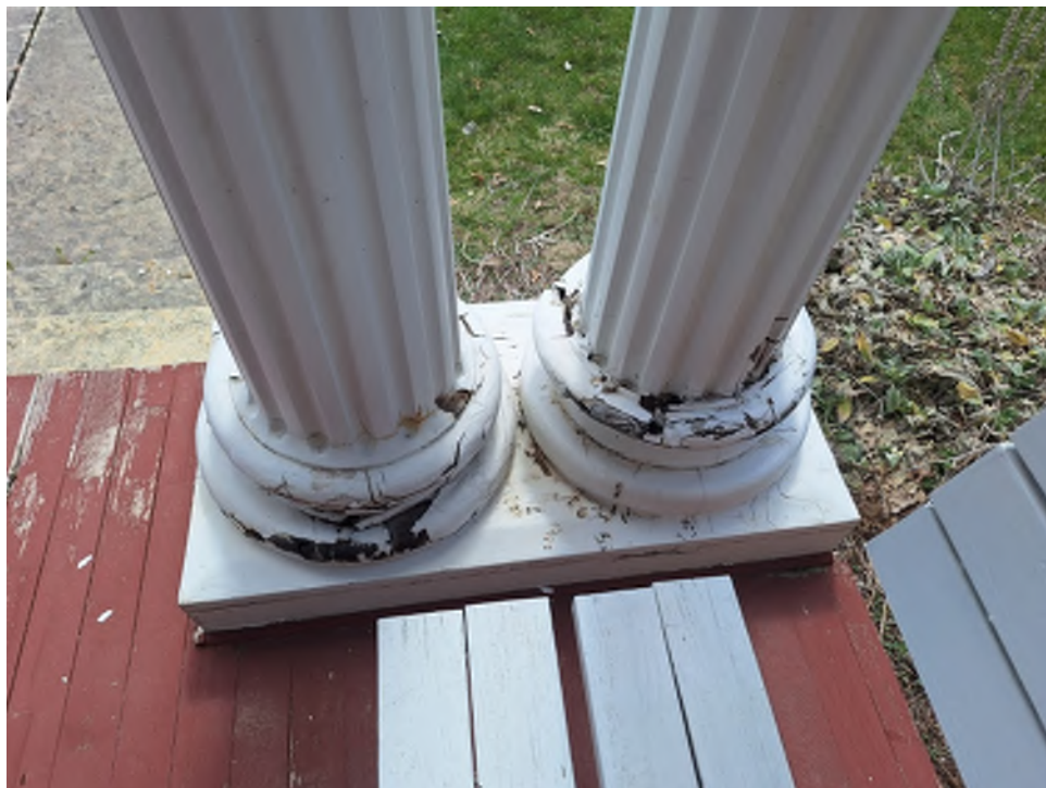
WEST COLUMN BASES - BACK SIDE
