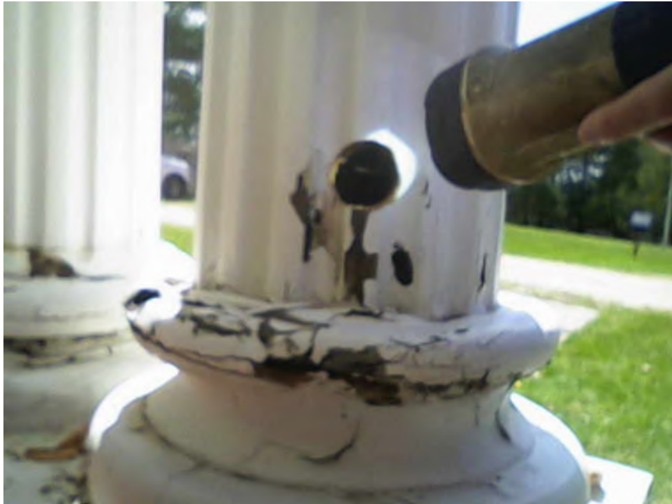
UPPER COLUMN EXPLORATORY HOLE
