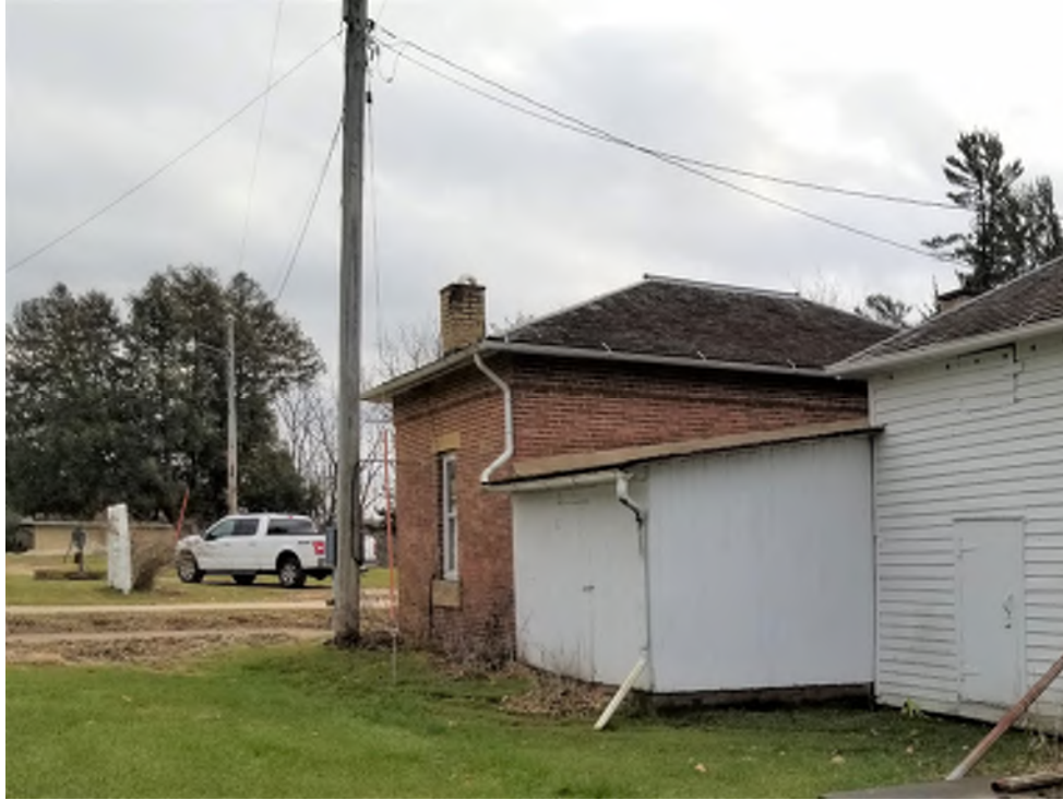
ELECTRICAL POLE NORTH OF WORKSHOP FOR OVERHEAD LINE
