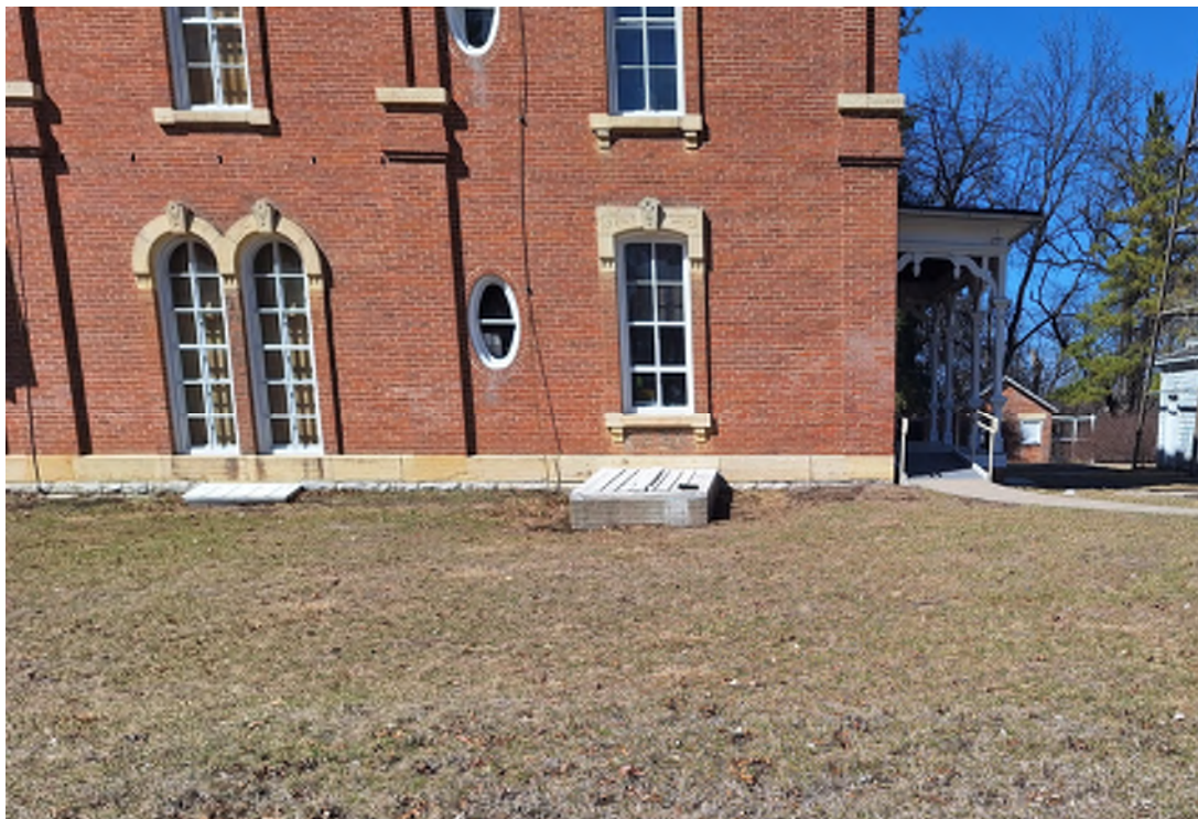
NORTHEAST SIDE OF MANSION AT GRADE SLOPE
