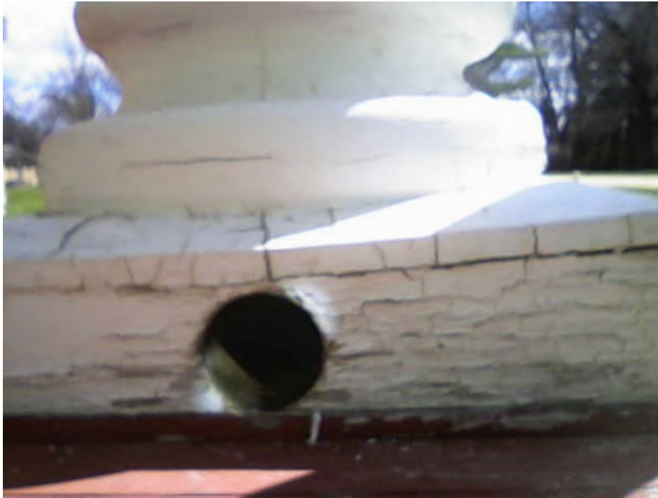
EXPLORATORY HOLE IN COLUMN BASES
