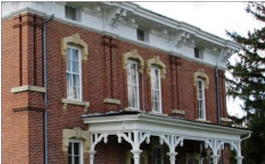
ELECTRICAL OVERHEAD LINE TO 2ND STORY WINDOW MASTHEAD
