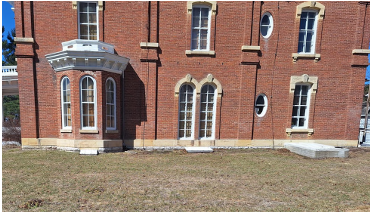
EAST SIDE OF MANSION AT GRADE SLOPE AND LIMESTONE TUCK POINTING
