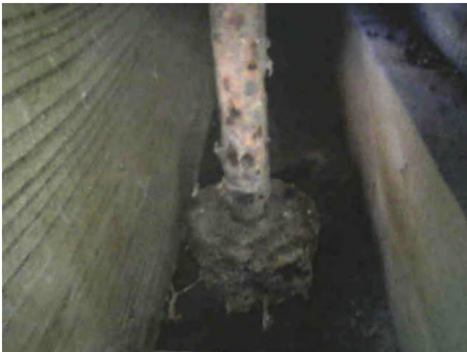
EXISTING TIE ROD BASE ANCHOR INSIDE COLUMN BASES
