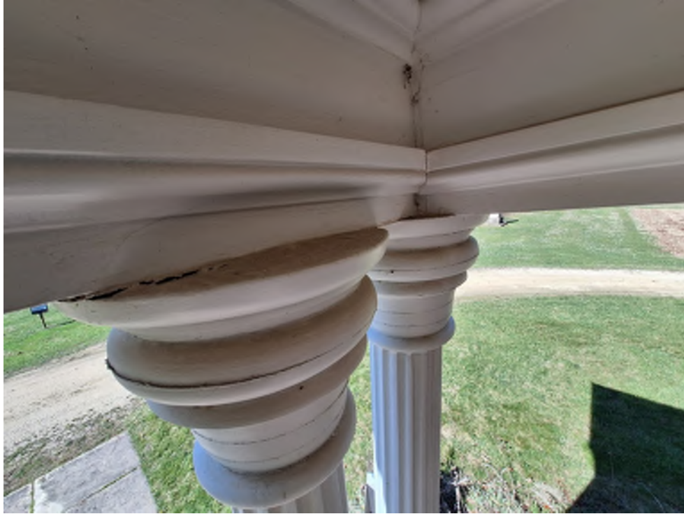
WEST COLUMN CAPITALS - TOP INSIDE
