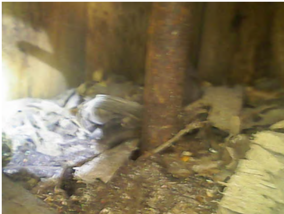
EXISTING TIE ROD INSIDE COLUMNS
