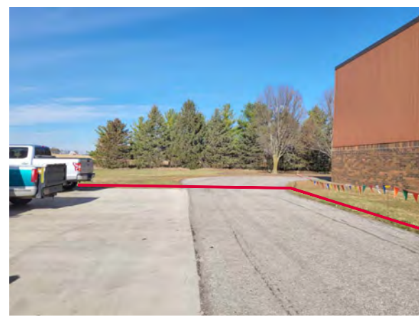
WEST SIDE OF ELEMENTARY SCHOOL
