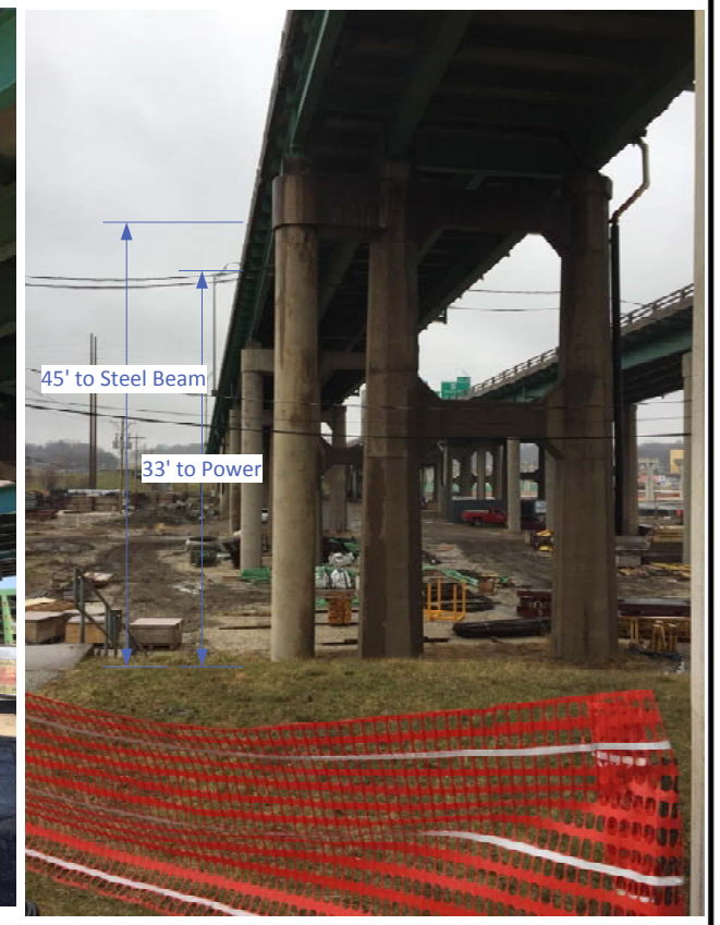
Pier 39 – ADSS above Power Lines
