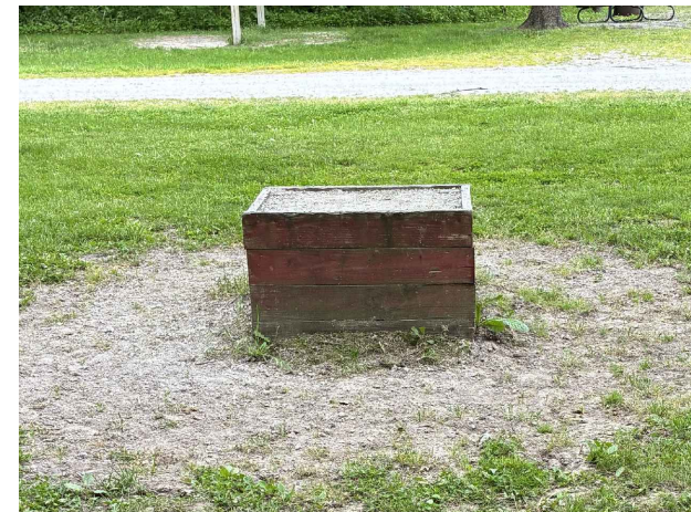
Existing Pit Latrines to be removed
