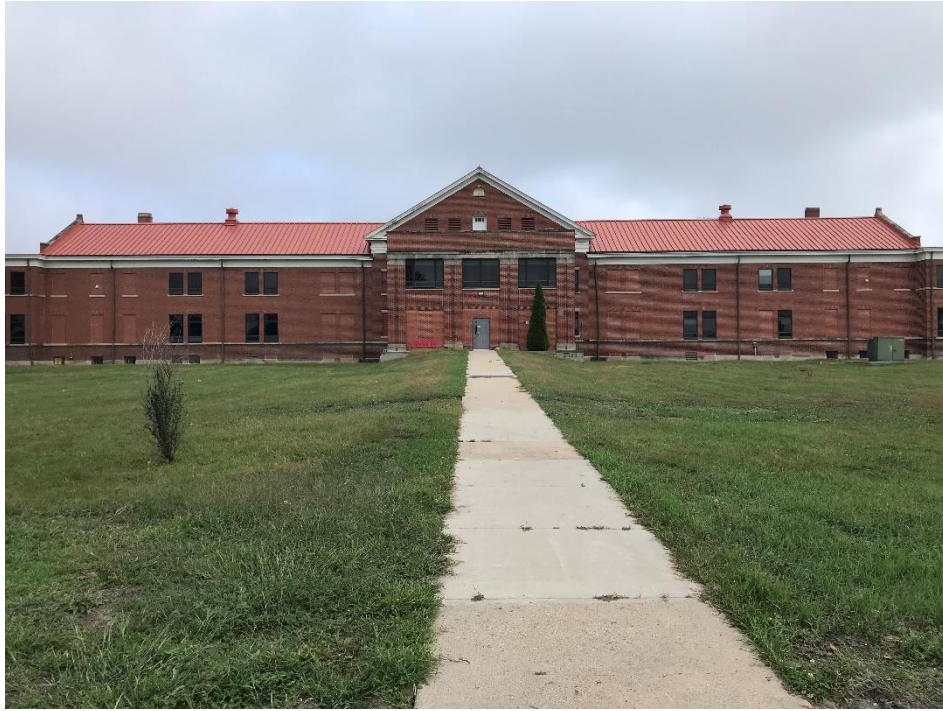
View of the Elmcrest Building.
