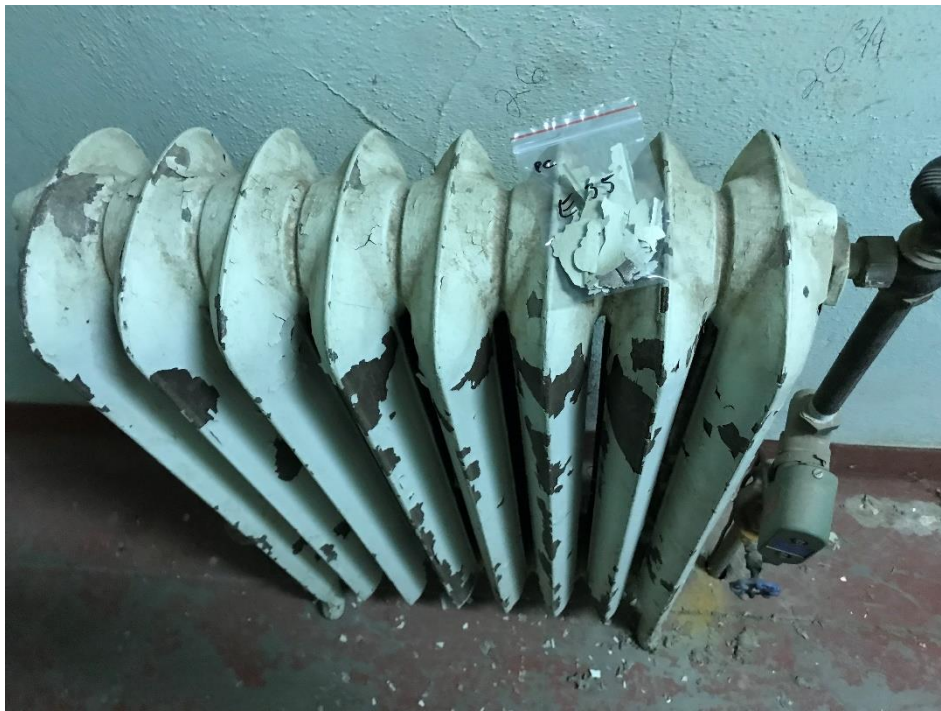
View of the Light Green Lead Containing Paint. (PC E 35, 0.36% Pb)
