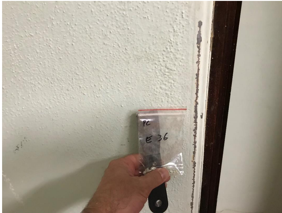
View of the Light Green Lead Based Paint. (PC E 36, 16% Pb)
