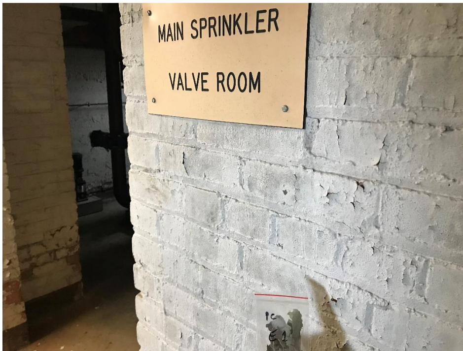
View of the White Lead Containing Paint. (PC E 1, 0.48% Pb)
