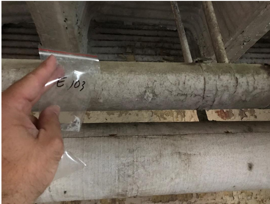
View of the Asbestos Containing TSI Run. (E 103, 10% Amosite & 10% Chrysotile)
