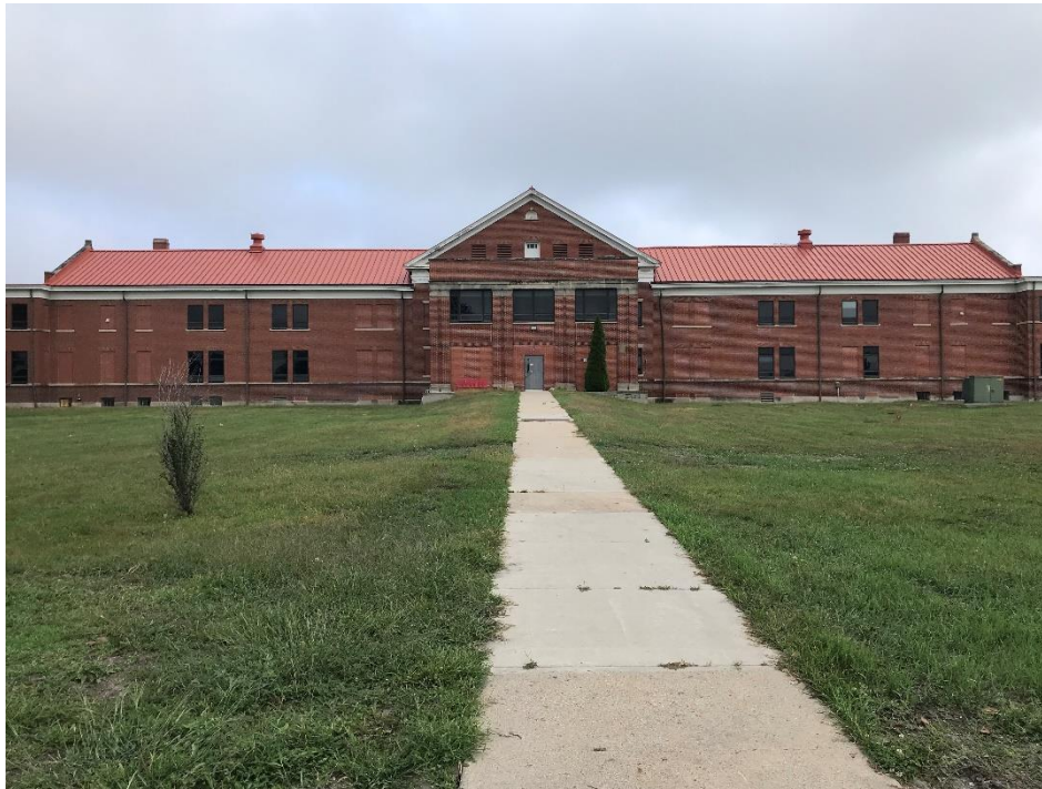
View of the Elmcrest Building.
