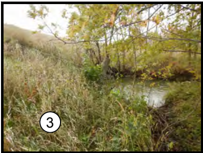
ICN STA. 87+48 AT CULVERT FLOW LINE FACING SOUTH
