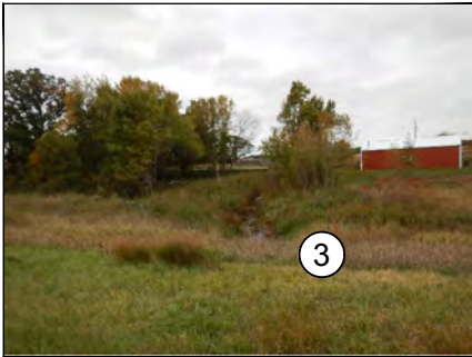
ICN STA. 183+77 LOOKING WEST FROM I-35 (SB)
