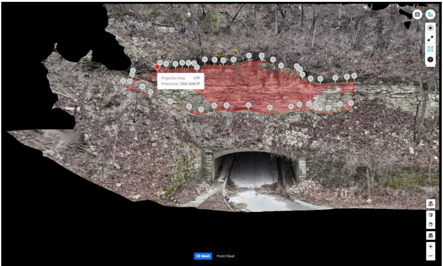
NE Entrance High Bluff Surface Area
