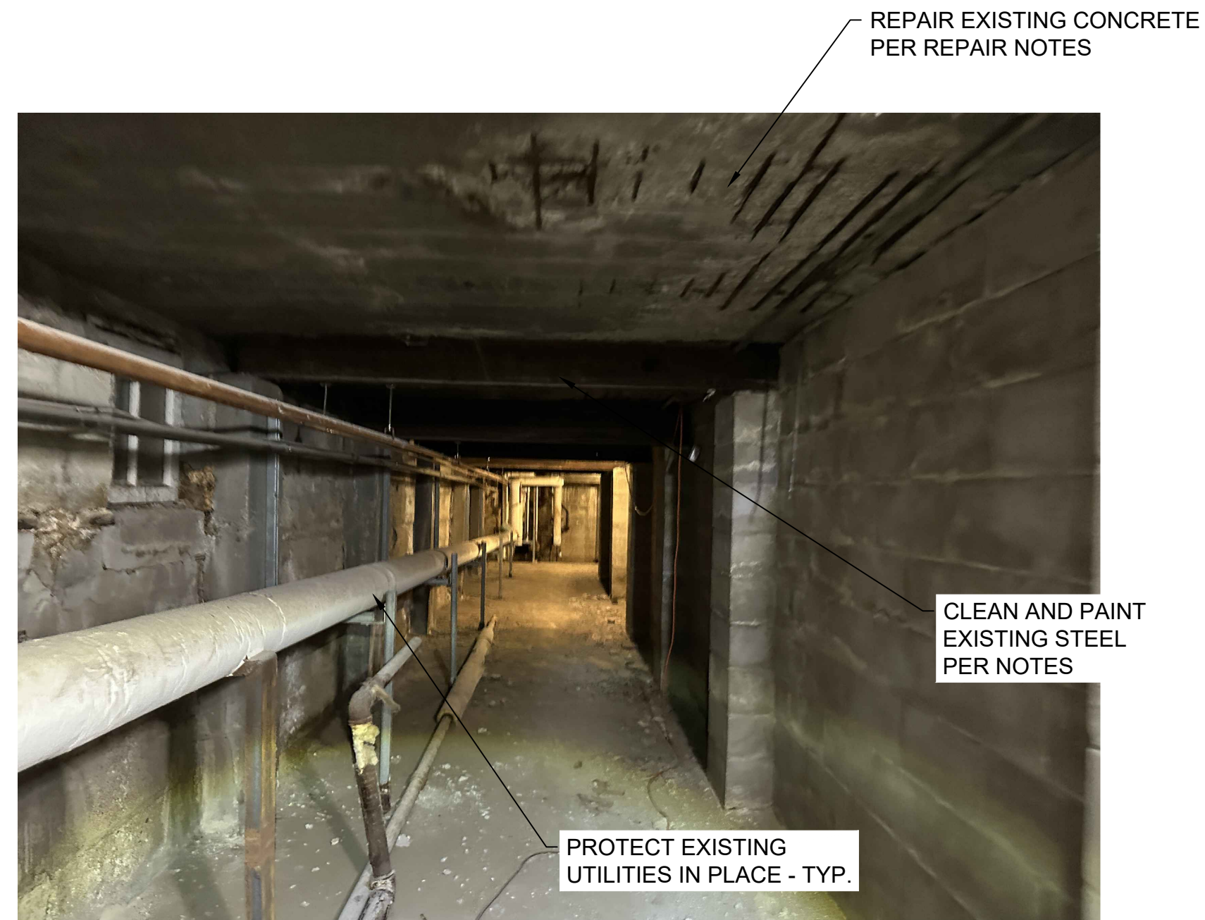
7 C14 TYPICAL TUNNEL SECTION PHOTO 7
