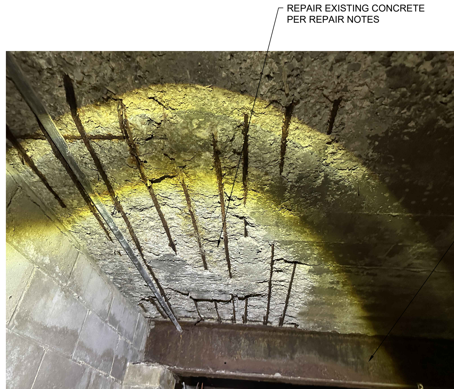
8 C14 TYPICAL AREA CONCRETE REPAIR PHOTO 8
