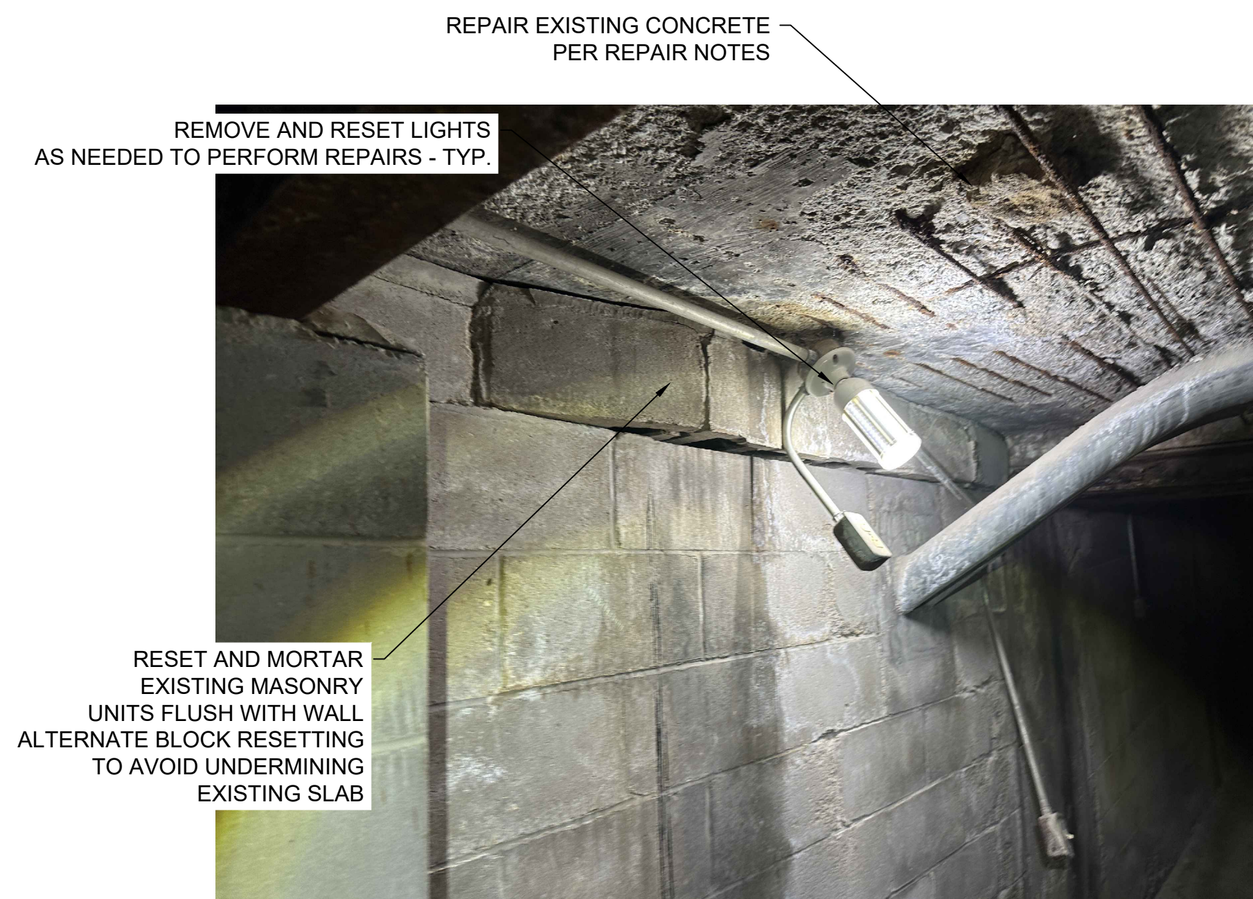
12 C14 AREA OF MASONRY REPAIR PHOTO 12
