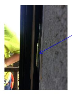
Daylight showing after primary seal (Exterior) was cut away.
