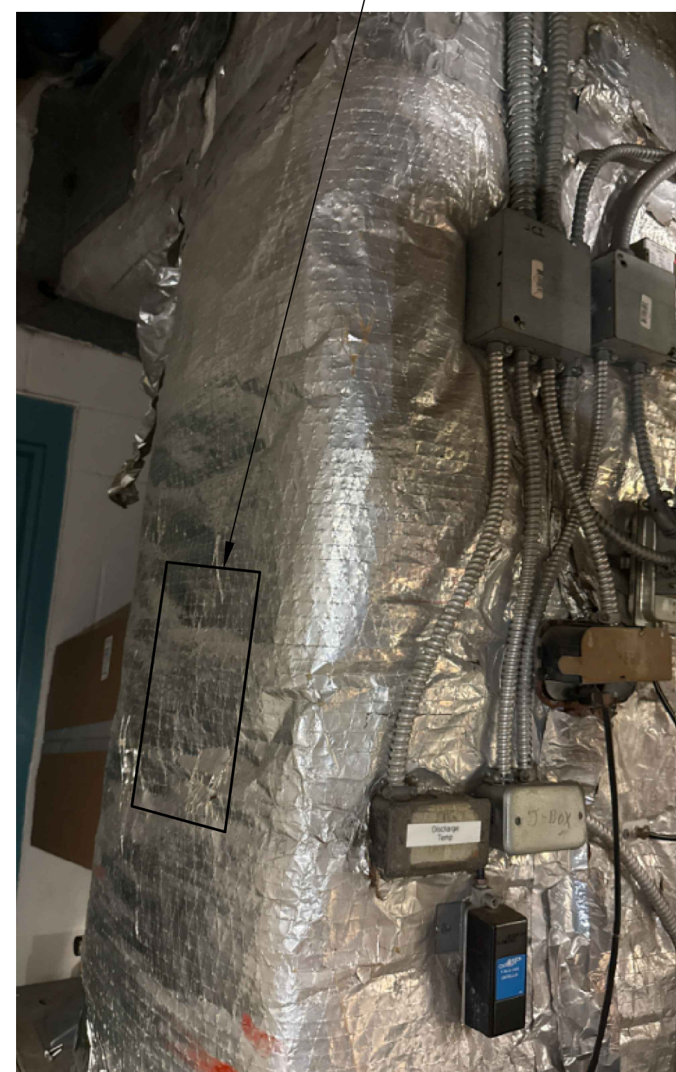
3 EXISTING MAU SUPPLY DUCT NOT TO SCALE
