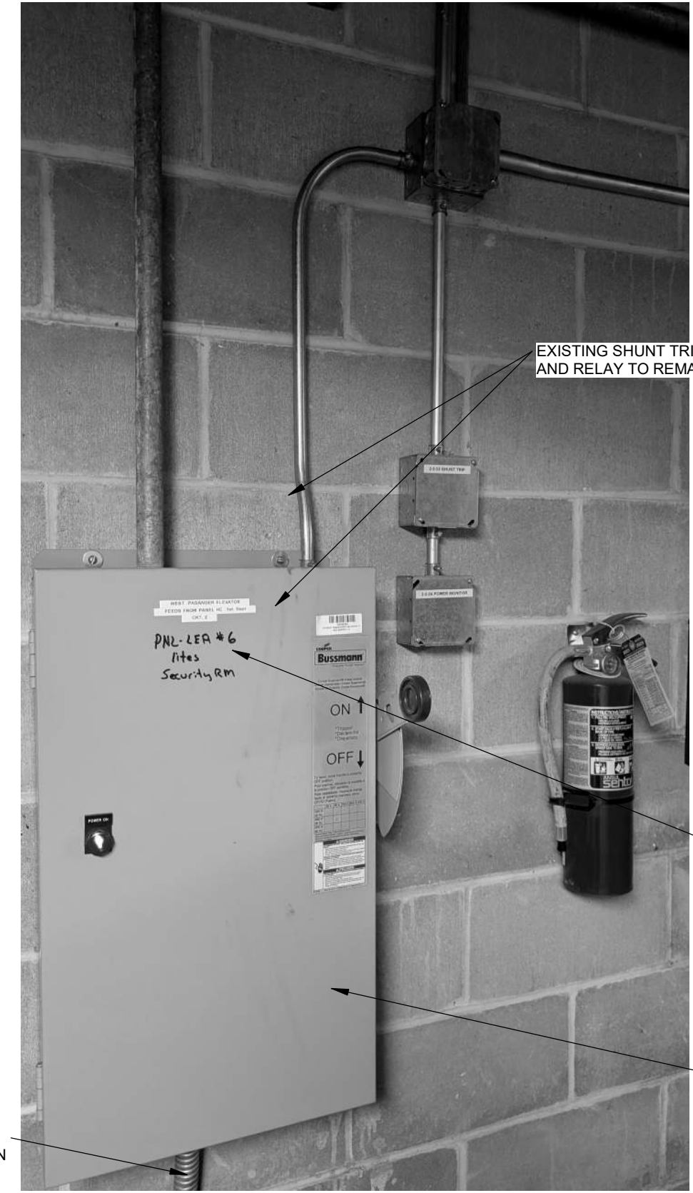
5 ELEVATOR 4 DISCONNECT 1/8" = 1'-0"
