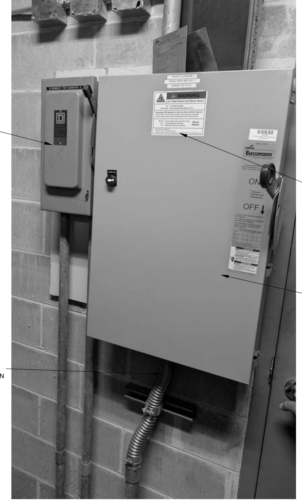
6 ELEVATOR 5 DISCONNECT 1/8" = 1'-0"
