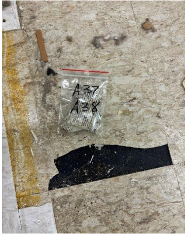
Photo #1 Sample 37 & 38 White 12 x 12 VFT and Black Mastic ( 2% & 6% Chrysotile ) Basement Room 013 Under White VFT.
