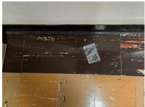
Photo #18 Sample A-65. Employee Home, Asbestos Containing 9" x 9" Floor Tile.
