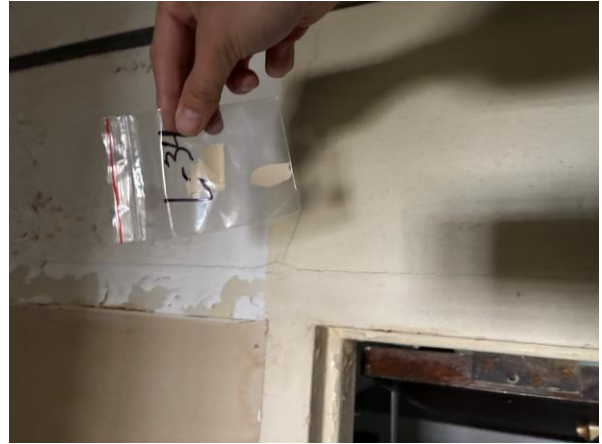
Photo #32 Sample L-34 – White Lead-based Paint on Plaster Wall in Larches 3 rd Floor.
