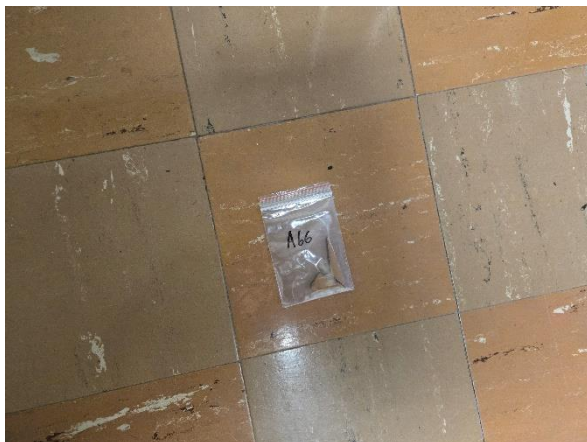
Photo #9 Sample A-66. Employee Home, Asbestos Containing 9" x 9" Floor Tile.
