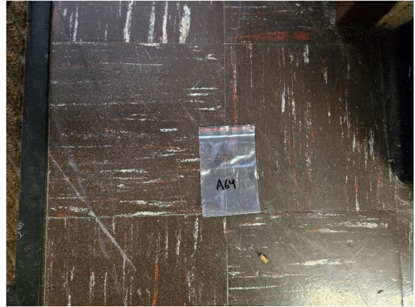
Photo #8 Sample A-64. Employee Home, Asbestos Containing 9" x 9" Floor Tile.
