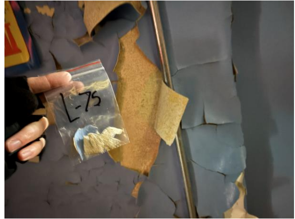
Photo #38 Sample L-76 – Blue Lead-based Paint on Concrete Wall in Hemlock 1 st Floor Central Wing.
