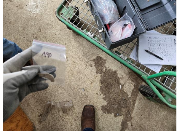
Photo #14 Sample A-90. Hemlock, Asbestos Containing Vinyl Sheet Flooring.
