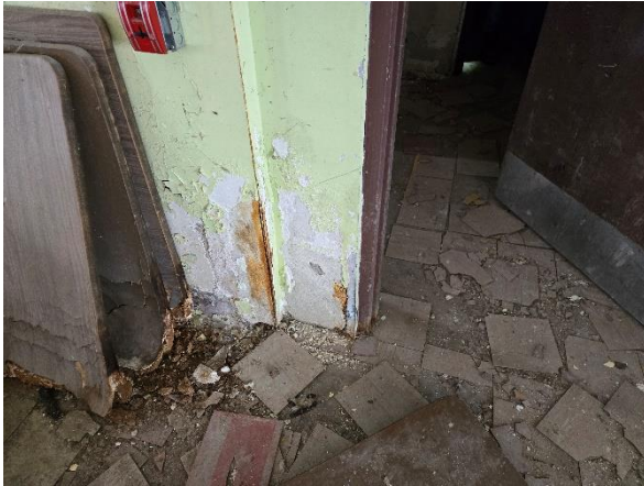
Photo #1 Sample A-7. Oak Hall, Asbestos Containing 9" x 9" Floor Tile and Black Mastic.
