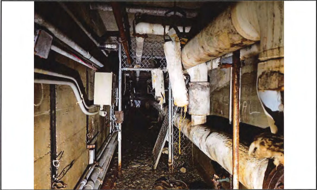
Photo 11: View of piping, conduits and fencing in the utility tunnel.
