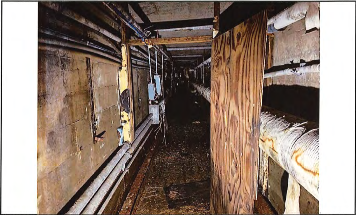
Photo 9: View of utility tunnel walls, fiberglass piping, conduits, and standing water.
