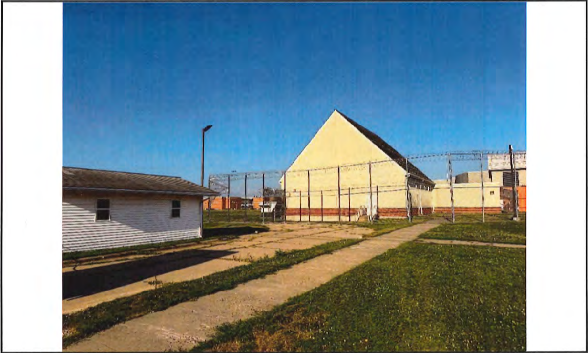
Photo 19: View of the sidewalk surface above the tunnel on the west side.
