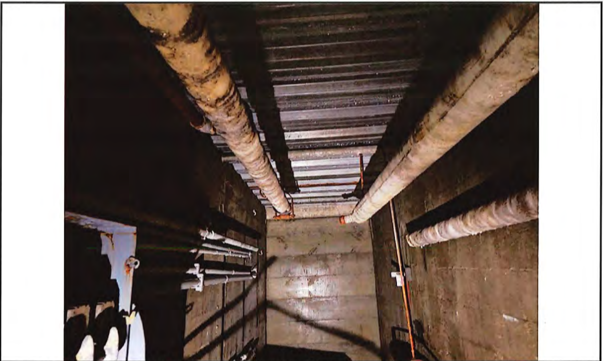
Photo 14: View of the pipes, concrete walls, and corrugated metal ceiling.
