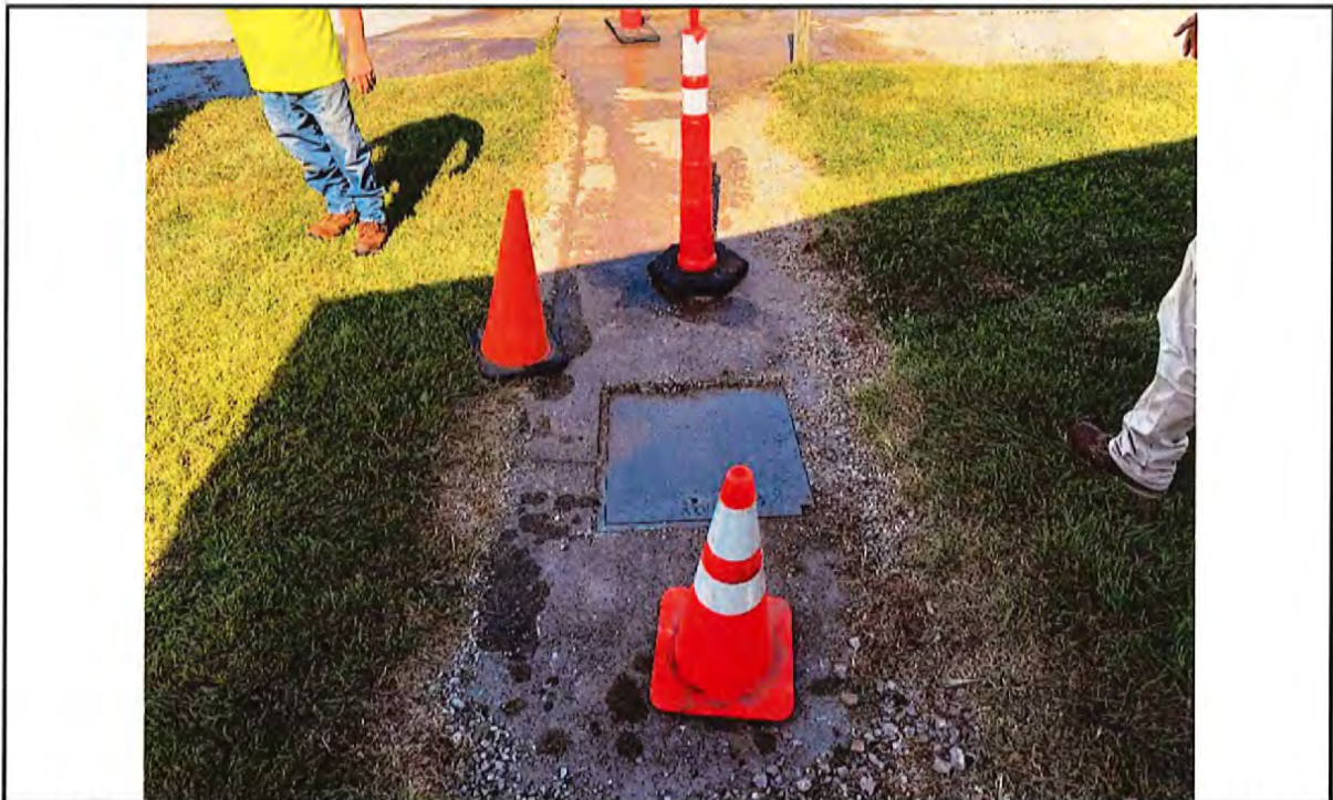
Photo 18: View of the sidewalk surface above the tunnel and the tunnel access port.
