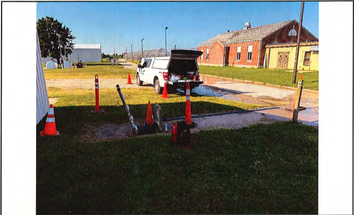
Photo 1: View of the entrance to the utility tunnel.
