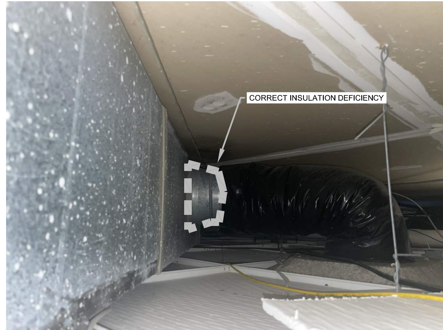
5 DUCT BRANCH RUN-OUT PHOTO NO SCALE
