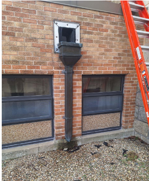
WEST SIDE LOWER ROOF SCUPPER & DOWNSPOUT
