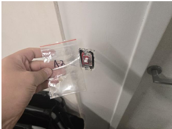
Photo #3 Non-ACM sample A-2. Drywall and joint compound found in
