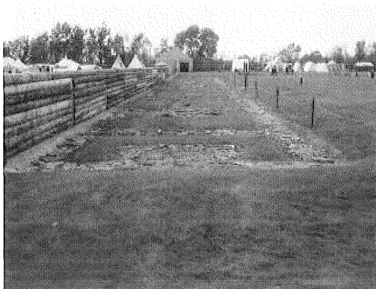
Figure 31. Photographs of Stockade Reconstruction in 2007, during the annual Rendezvous. Upper: facing southwest, toward the Powder Magazine (Contributing Structure #1). Lower: facing west, along the south wall of the Palisade, toward the Southwest Blockhouse (Contributing Structure #2). Foundations are those of the South Barracks (originals on file, Iowa Office of the State Archaeologist, Iowa City).
