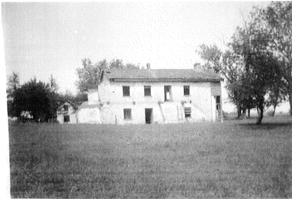
Figure 18. Historical photographs of the North Barracks. Upper: probably between 1912 and 1919, facing northeast (original on file State Historical Society of Iowa, reproduced in Whittaker 2006d:33). Lower: dated August 2, 1935, facing northwest (original on file, Fort Atkinson Museum, reproduced in Whittaker 2006d:36).
