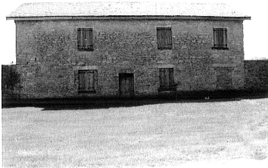
Figure 20. Photographs of the North Barracks in 2006. Note the Stone Wall (Contributing Structure #3) that extends to the east and west of the building. Upper: facing north. Lower: facing south (from Whittaker 2006:40).
