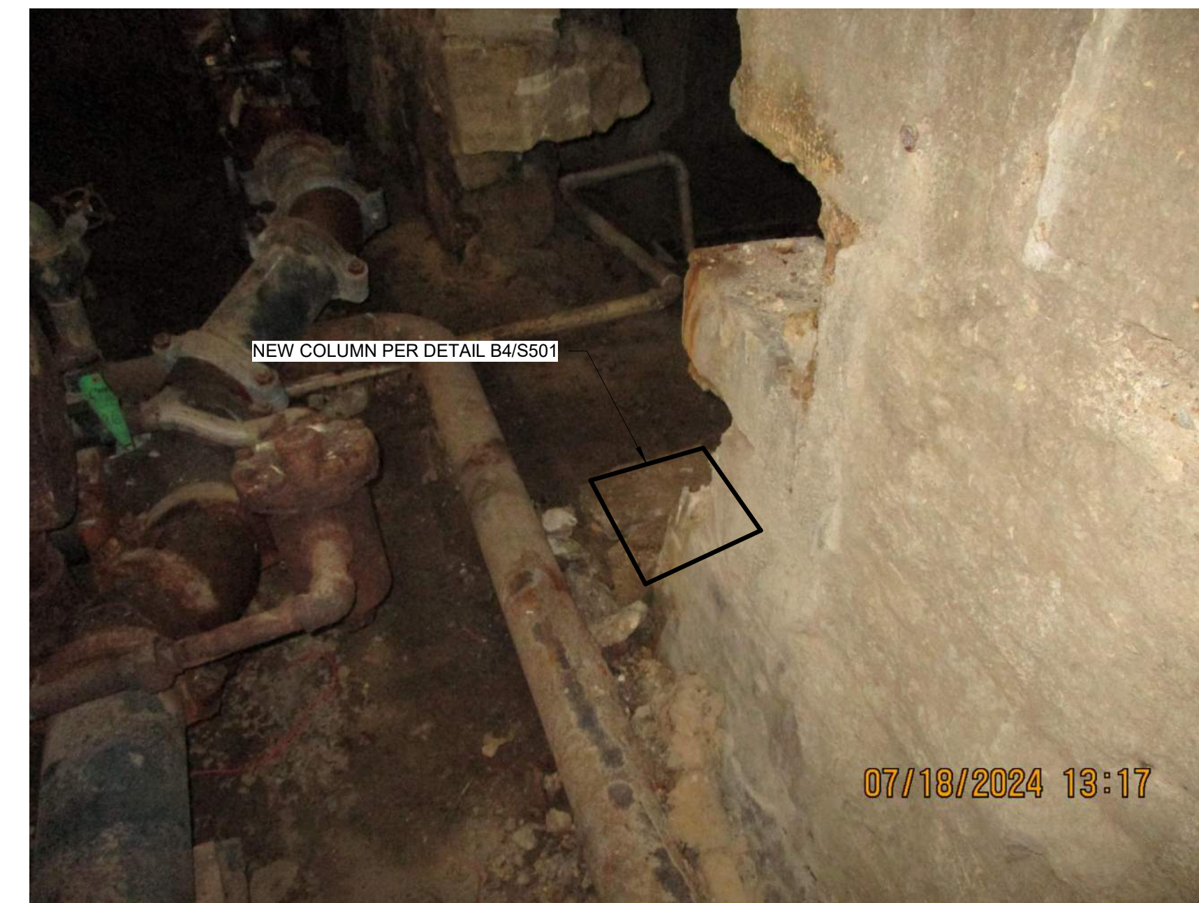
(E4) SOUTH TUNNEL - PHOTO 3 (STA 3+05) 1 1/2" = 1'-0" 0" 1'
