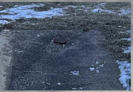
VIEW OF DRAIN INTAKE FROM WEST, LOOKING EAST.
