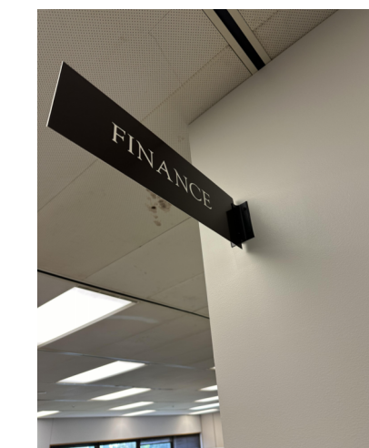
* EXISTING DIRECTIONAL, INFORMATIONAL, AND ROOM SIGNAGE TO BE REMOVED, SALVAGED, & REINSTALLED, TYP. SEE PHOTO ABOVE FOR REFERENCE.
