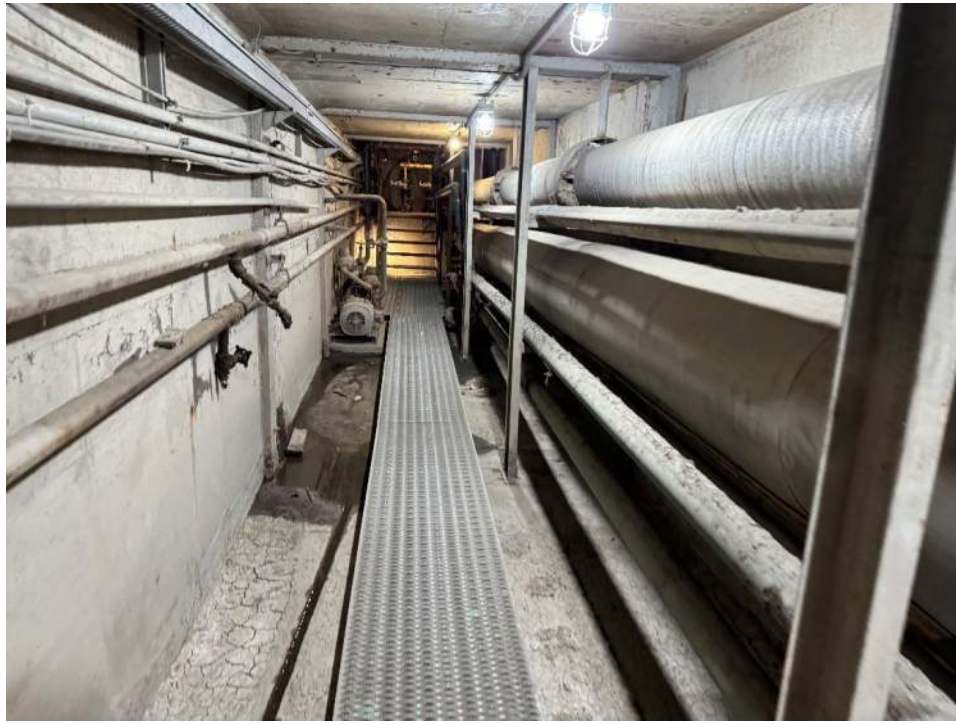
View of the Powerhouse Tunnel Entrance.
