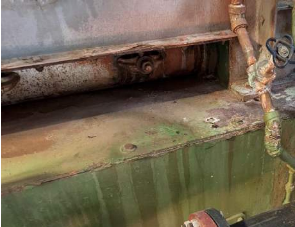
Photo #13 Sample PPC-4. Green lead-based paint on south coal burner in north room.
