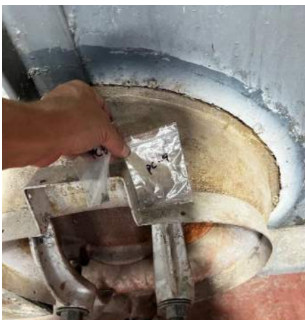
Photo #17 Sample PC-9. Silver paint on metal tube end of boiler #2
