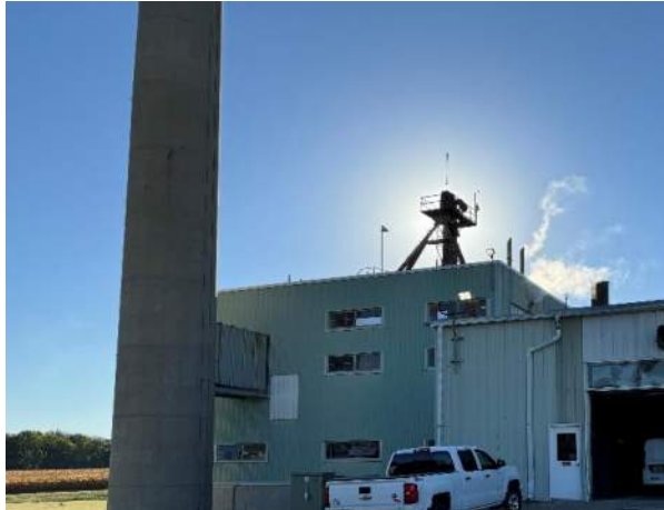
Photo #1 View of the Powerhouse.
