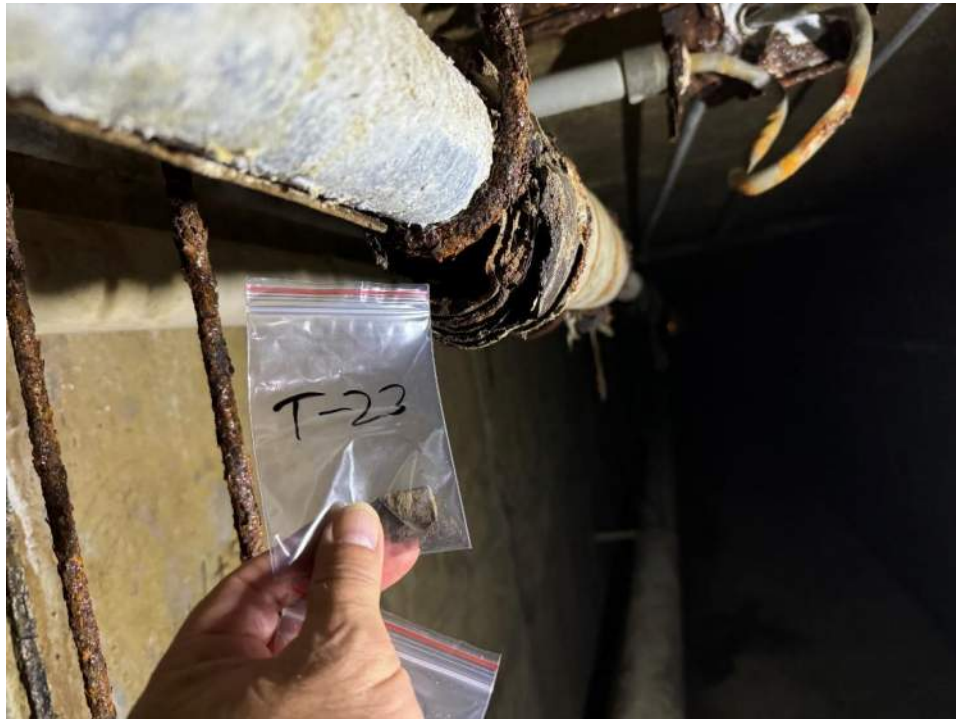
View of the Asbestos Containing 2" Pipe Run. (T-23, 50% Chrysotile)
