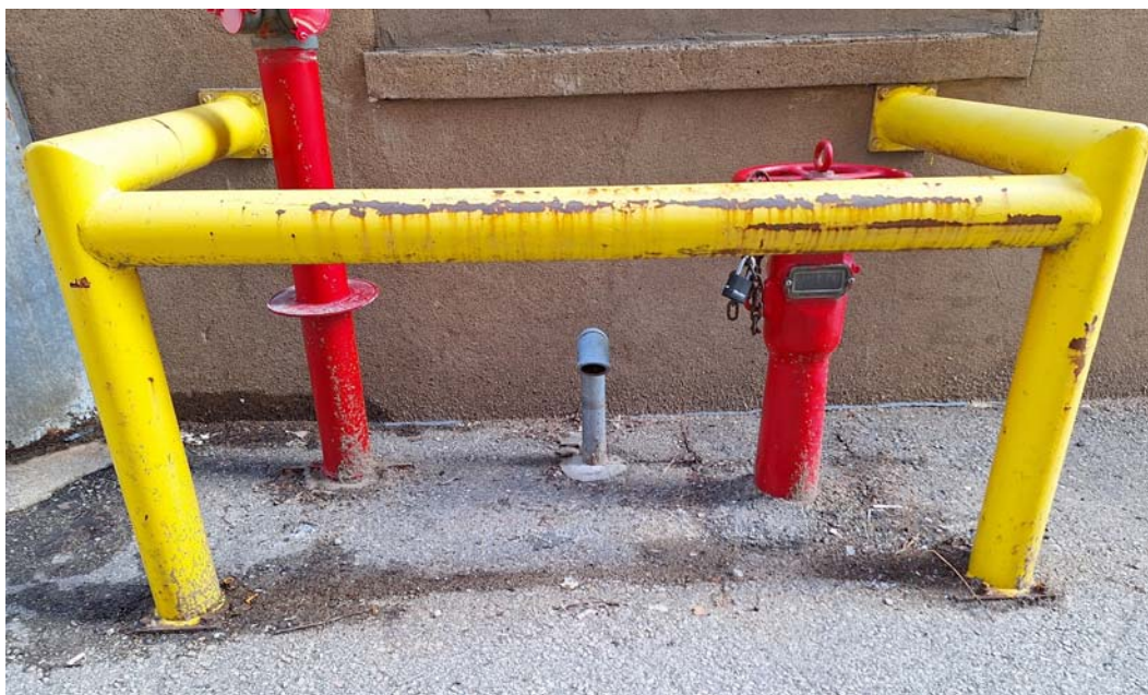
SPRINKLER PIPES & BOLLARD STANCHION
