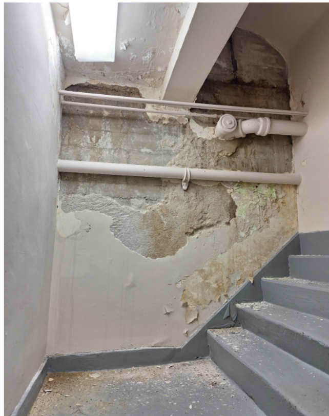
BASEMENT PLASTER REPAIRS
