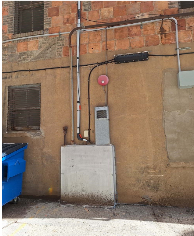
ALLEY WALL - NORTH CONCRETE PIER
