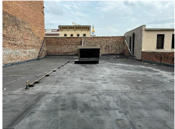
Photo #8 Overview of roof area.
