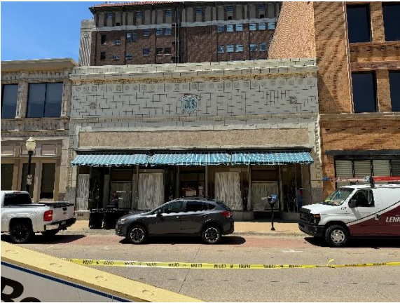
Photo #1 Looking at DPP Building.
