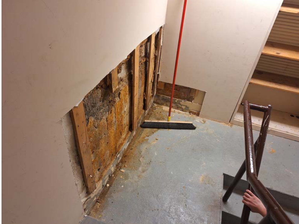
STAIRWAY DRYWALL REPAIRS
