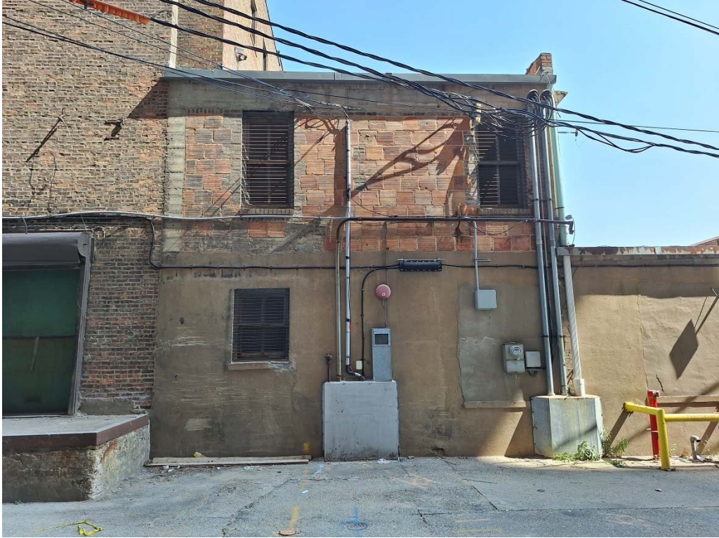
ALLEY EXTERIOR WALL - NORTH HALF
