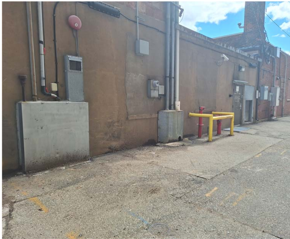
REAR WALL OF BUILDING
