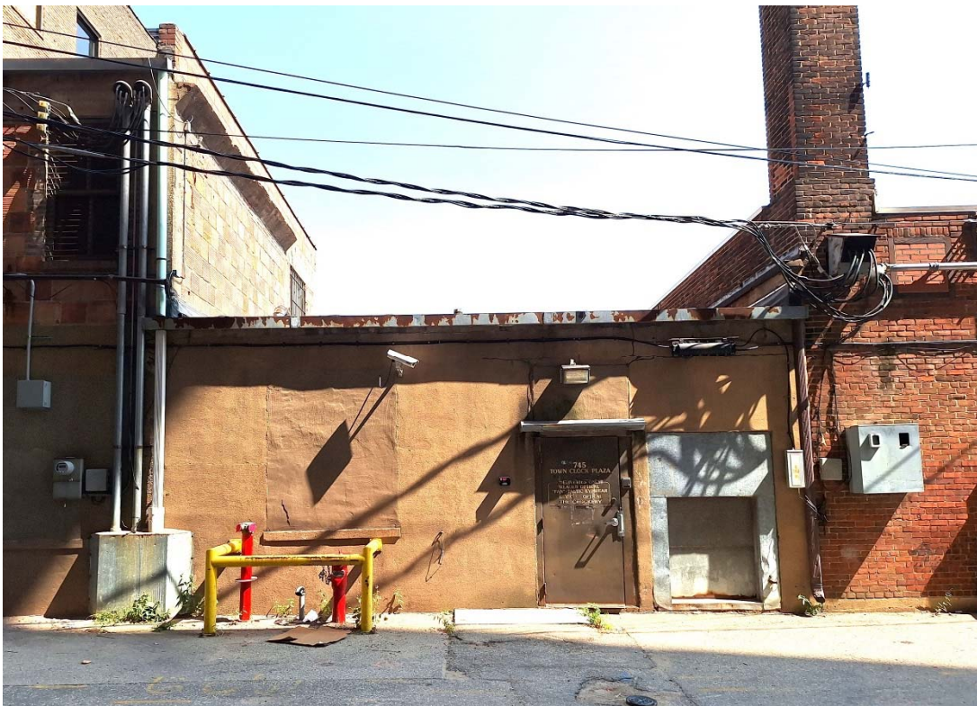
ALLEY EXTERIOR WALL - SOUTH HALF
