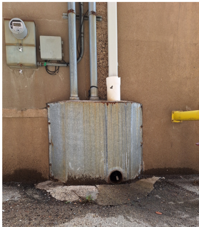
ALLEY WALL - SOUTH CONCRETE PIER
