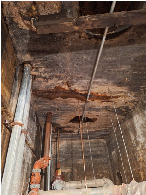
BASEMENT UTILITIES UNDER ALLEY
