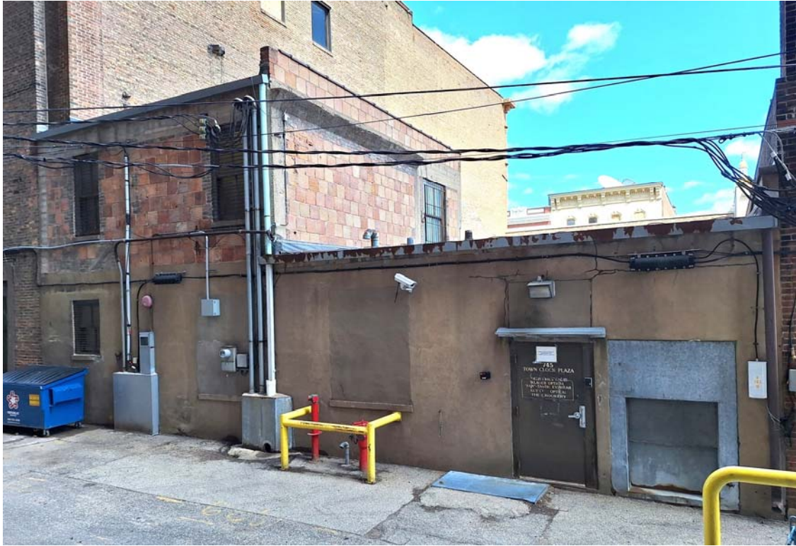
REAR WALL OF BUILDING
