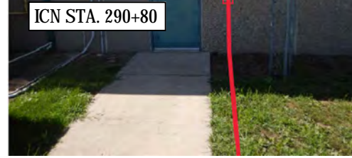
ELECTRICAL ROOM - LOOKING WEST
