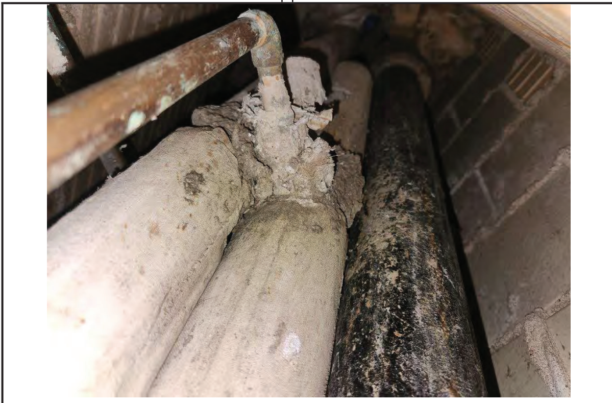
Photo 8: View of vertical runs of pipe insulation.
