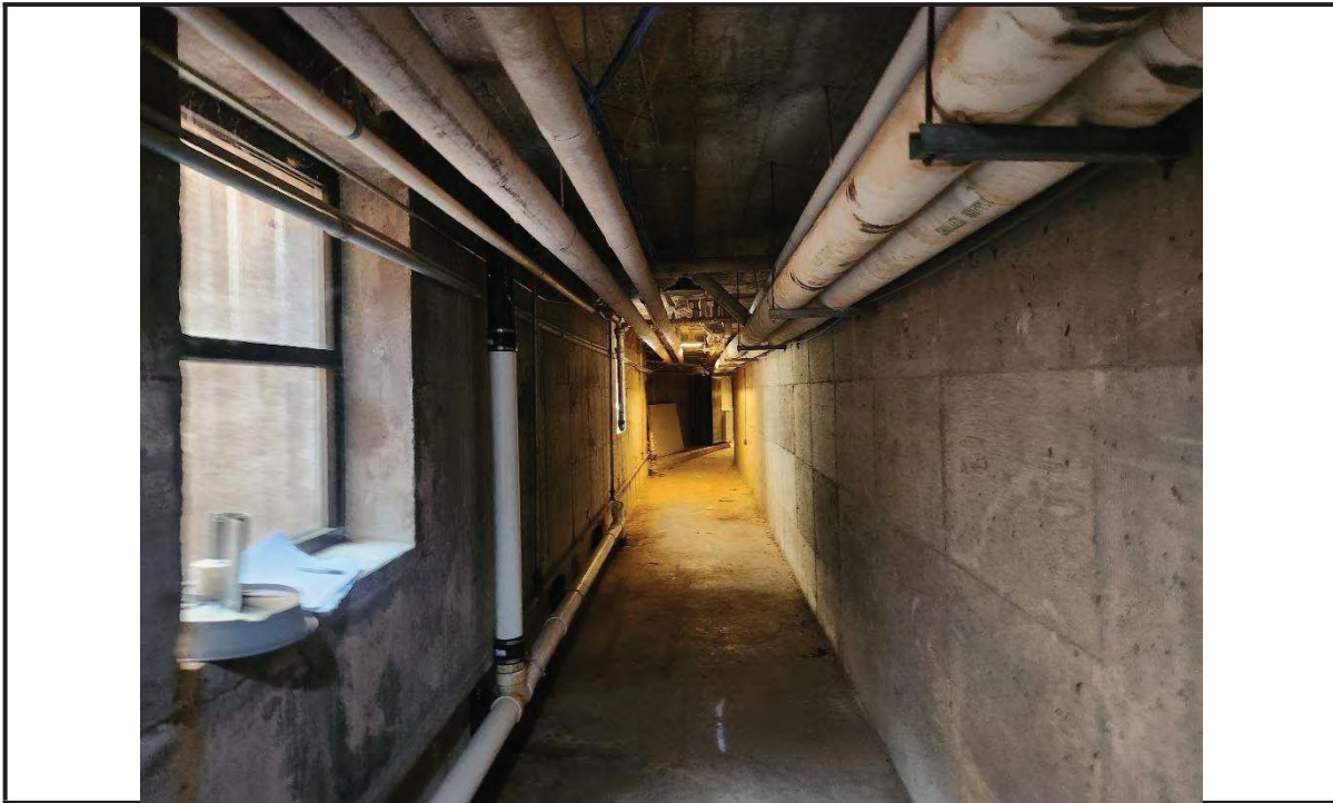
Photo 1: View of ACM linear pipe runs in Basement Area B.
