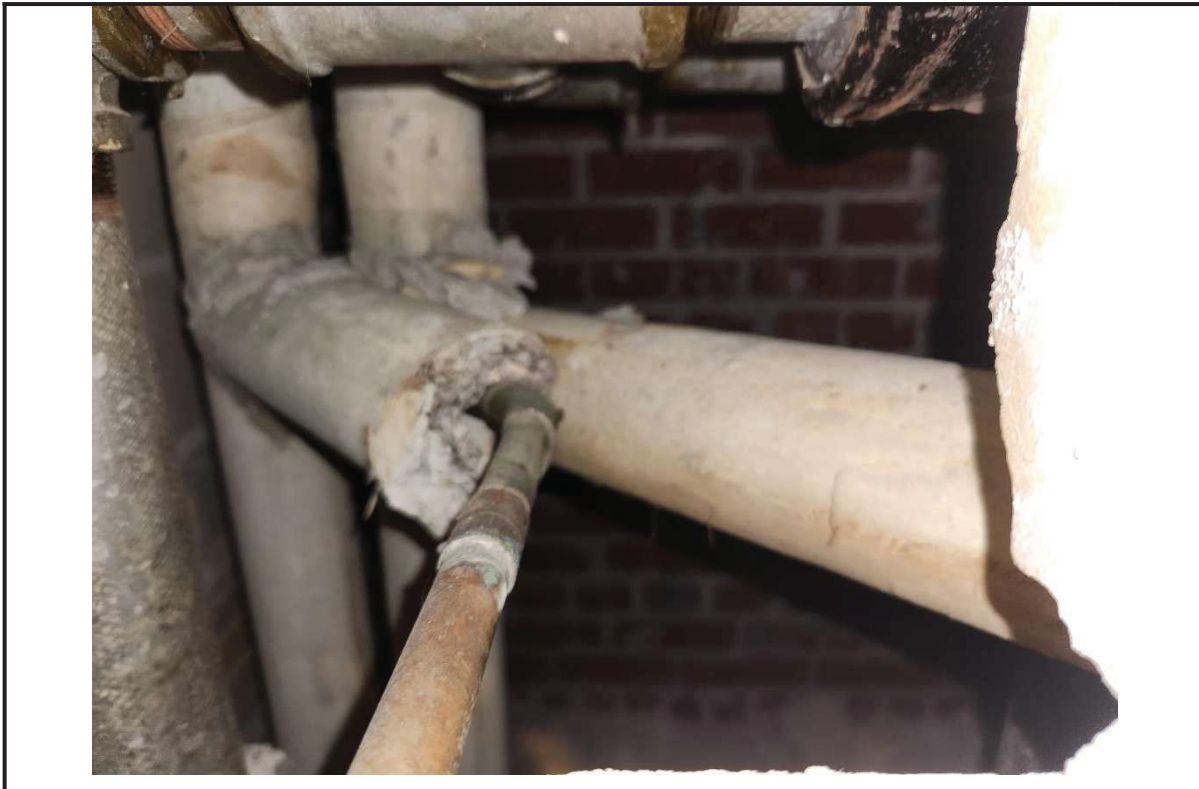
Photo 7: View of ACM pipe insulation in 3 rd Floor Area A.
