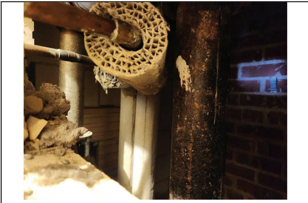
Photo 4: View of ACM paper pipe insulation on 3 rd Floor Area A.
