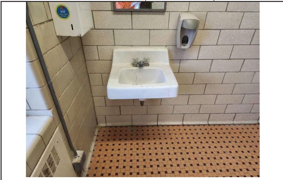
Photo 12: View of typical ceramic block wall and sink fixture.
