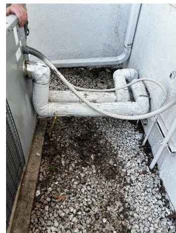
Photo #6 Paint Sample PC-1 – White Paint on Exterior Stucco.
