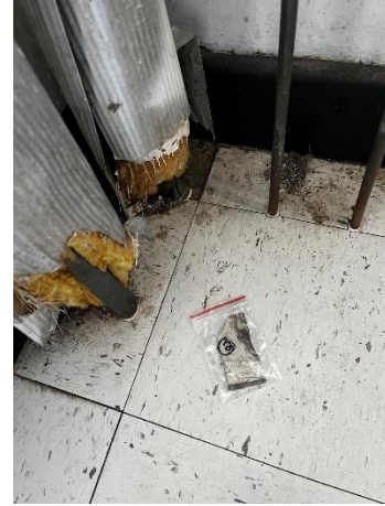
Photo #2 Samples #2&3 – 12"x12" Floor Tile & Brown Mastic – House A Stair Landing
