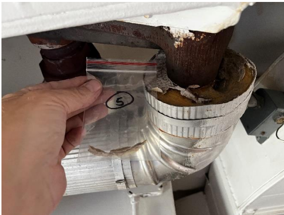
Photo #3 Sample #5 – White Pipe End Sealant – House A Stair Landing
