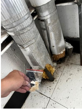
Photo #1 Sample #1 – Pipe Insulation under Metal Jacket – House A Stair Landing
