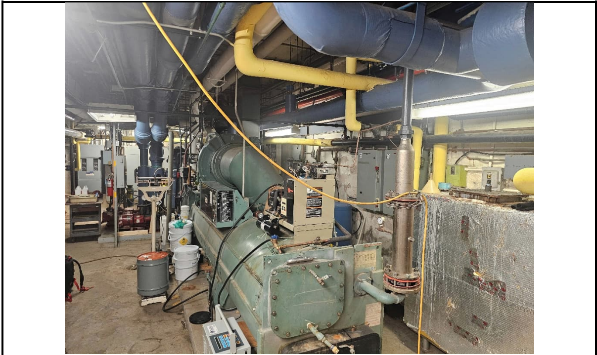
Photo 1: View of the project area.
