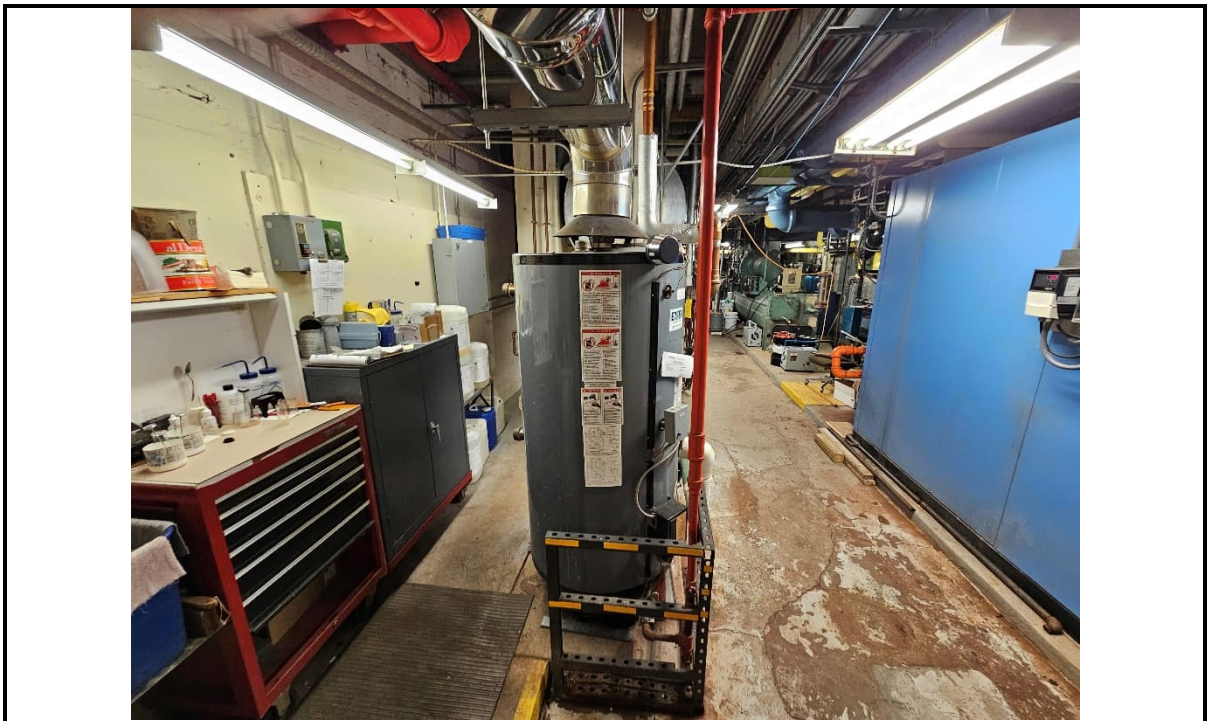
Photo 4: View of the project area.
