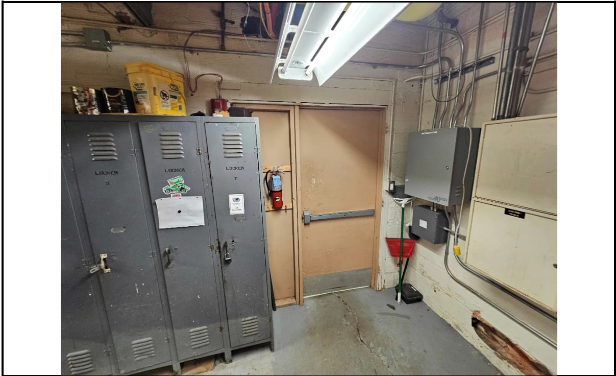
Photo 3: View of the project area.
