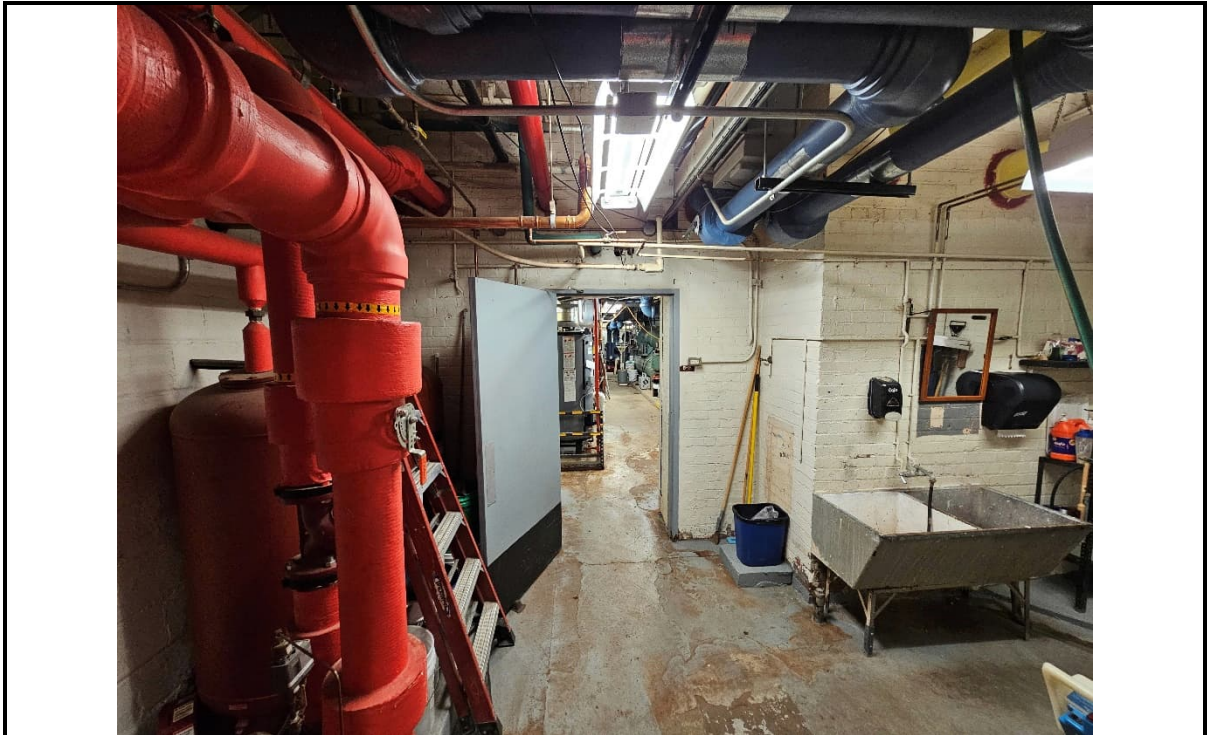
Photo 2: View of the project area.
