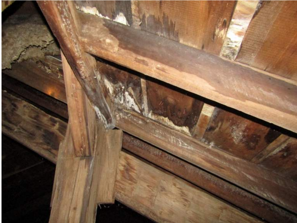
ATTIC RAFTER REPAIRS
