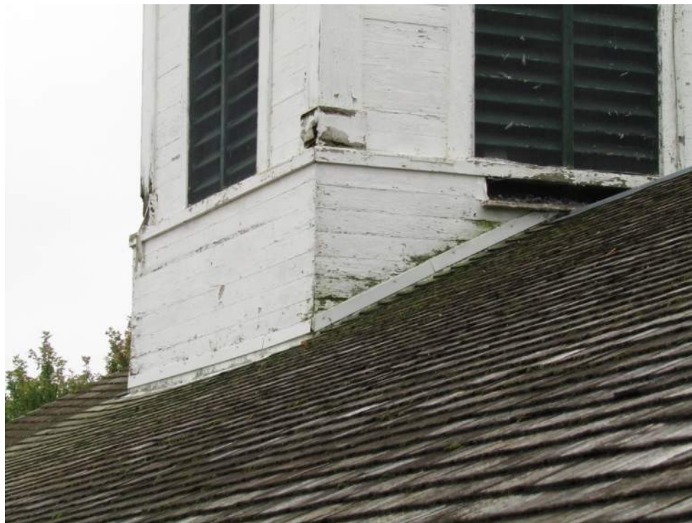
NORTHEAST STEEPLE BASE
