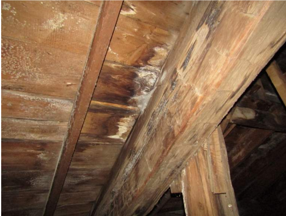
ATTIC RAFTER REPAIRS
