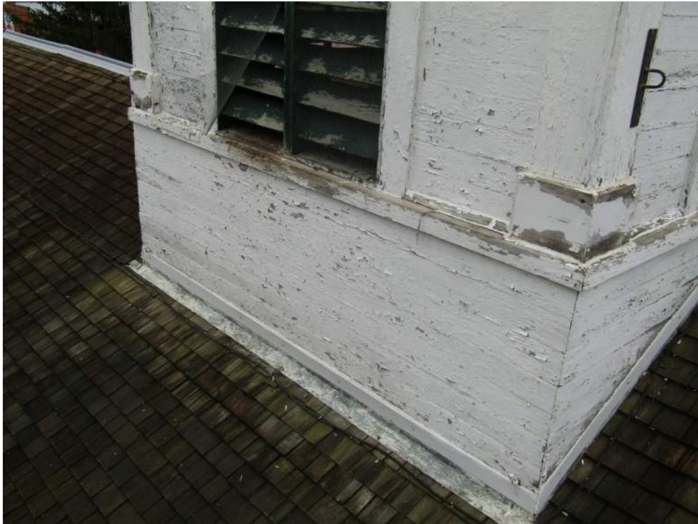
SOUTHWEST STEEPLE BASE
