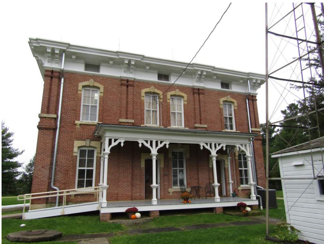
VIEW OF NORTH
