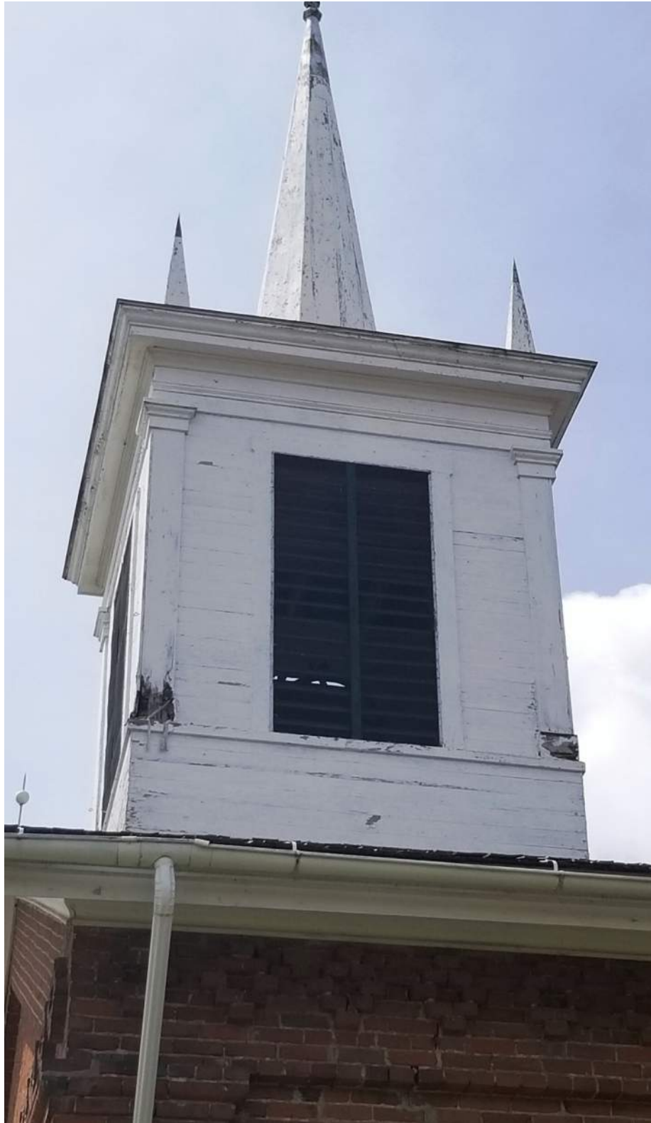
VIEW OF EAST STEEPLE WALL
