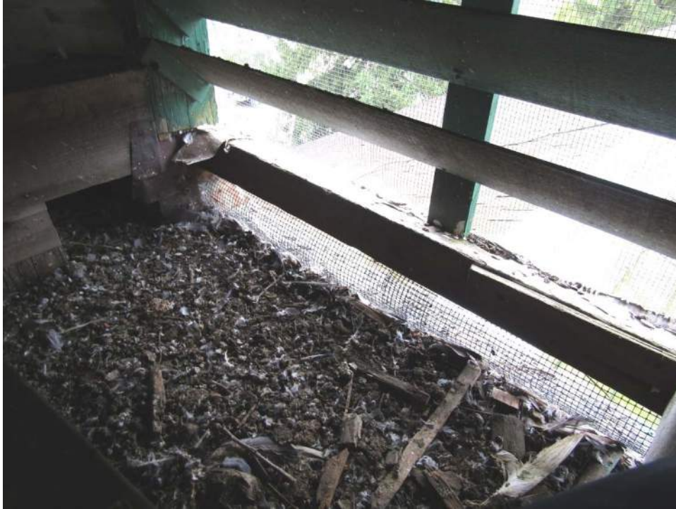
NORTH SIDE BELL TOWER FLOOR SCUPPER
