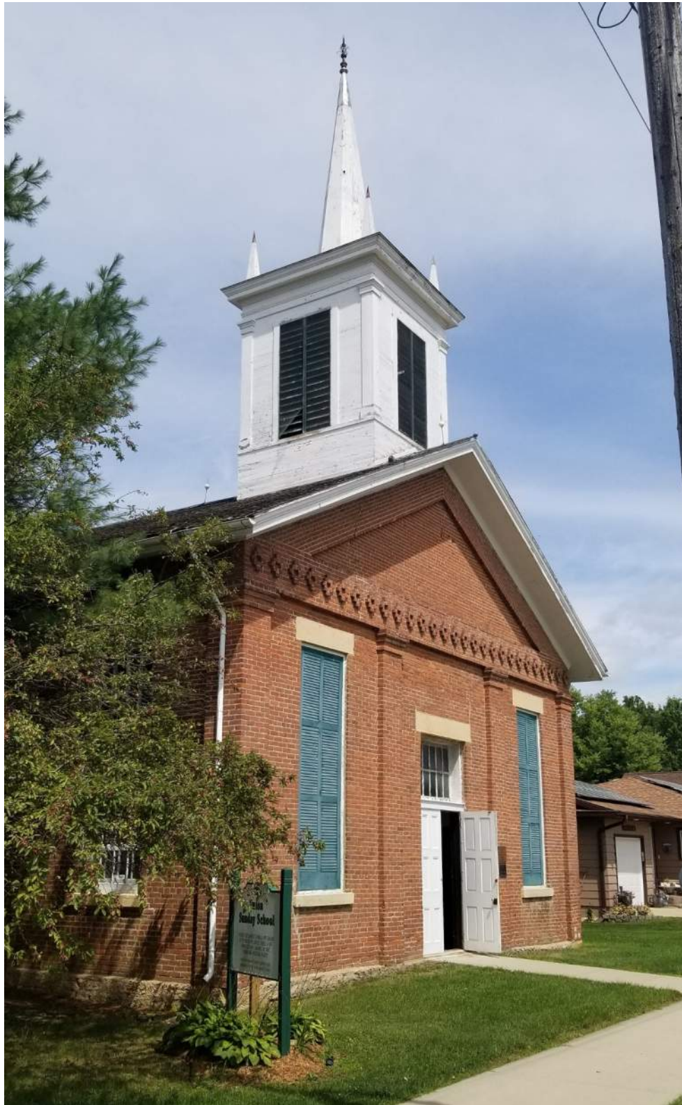
VIEW OF SOUTH ENTRANCE FROM WEST
