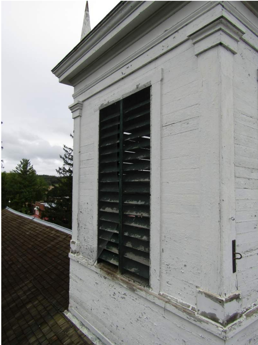
WEST FACE STEEPLE
