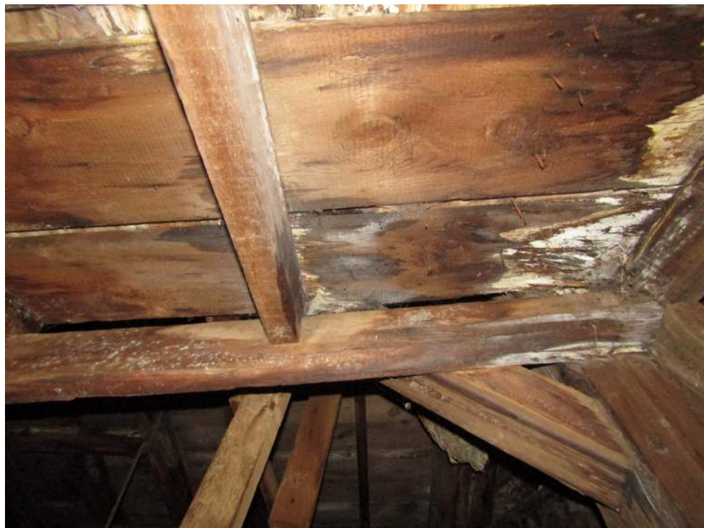
ATTIC RAFTER REPAIRS
