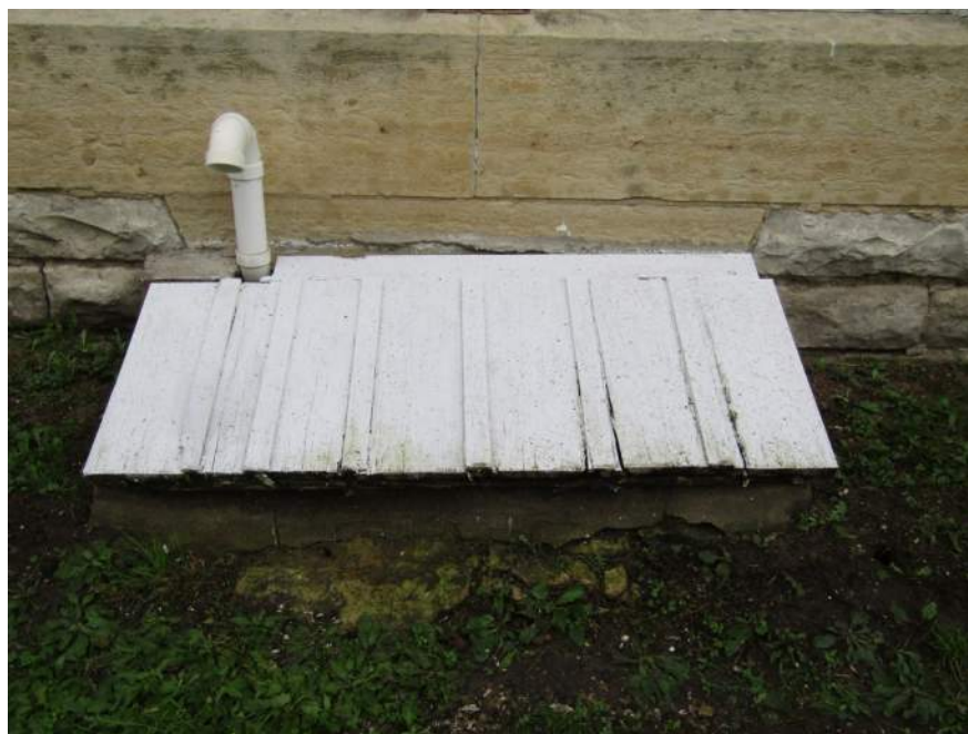
BASEMENT WINDOW WELL COVER AT WC-4
