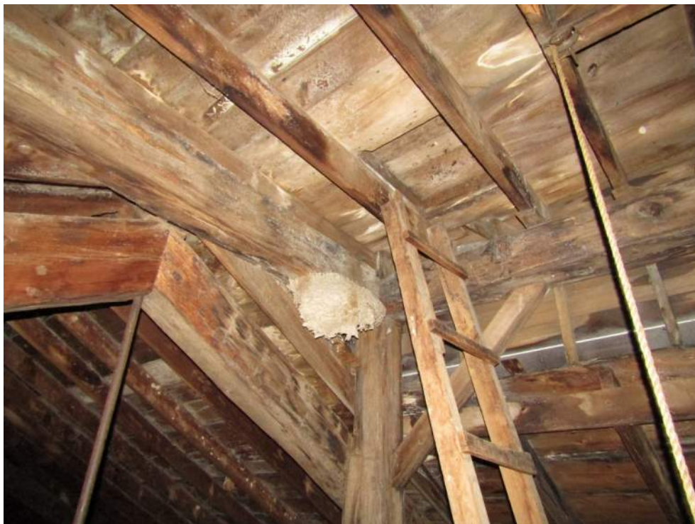
STEEPLE ACCESS NEAR RAFTER REPAIR AREA
