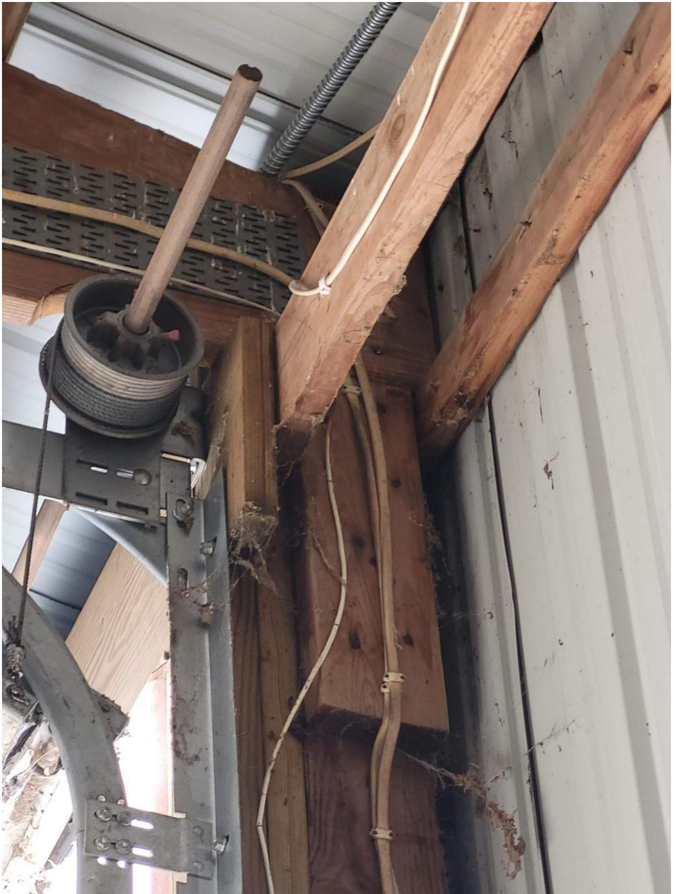
Header on 18'W door that needs an additional 2'X12' added. See ERI section for more details. Base bid item.
