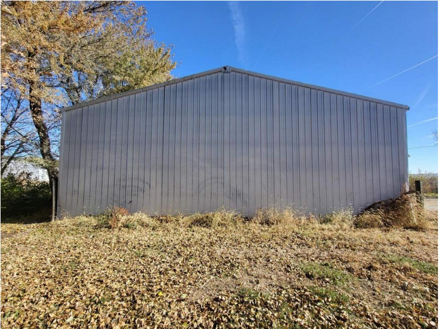
Side view, looking east. Remove and replace all existing metal siding, roofing and trim work with like style 29-guage ribbed tin. Dispose of off-site. See ERI section for more details. Base bid item.
