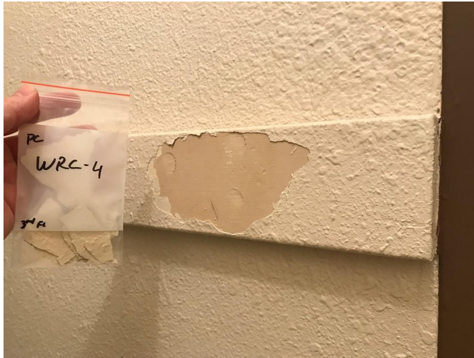
View of off-white paint on walls on 3 rd floor. (0.0098% wt)
