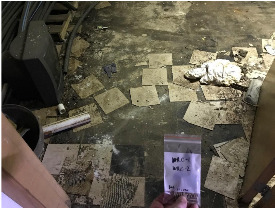
View of Beige 9" x 9" Vinyl Floor Tile in Basement (WRC-1, 5% Chrysotile)
