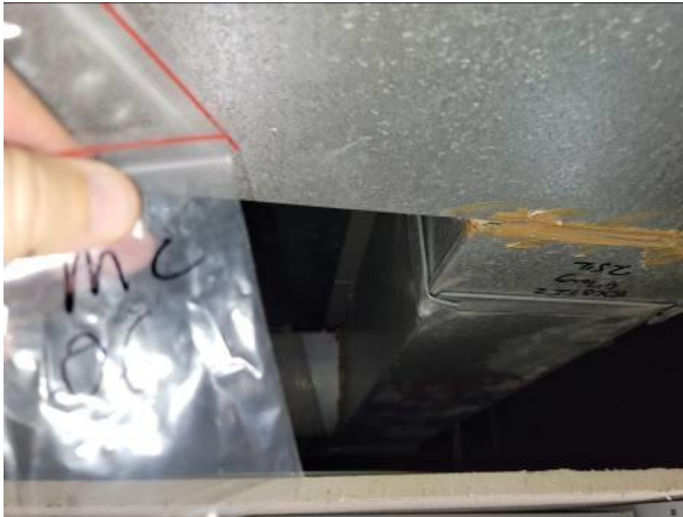
View of Tan Duct Sealant (2% Chrysotile)
