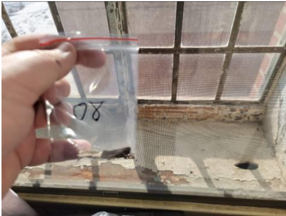
View of White Window Glazing (2% Anthophyllite 2-3% Chrysotile)
