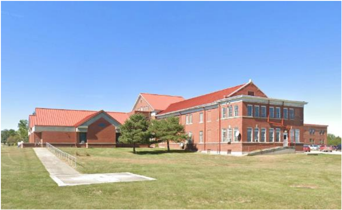
View of the Woodward Medical Center
