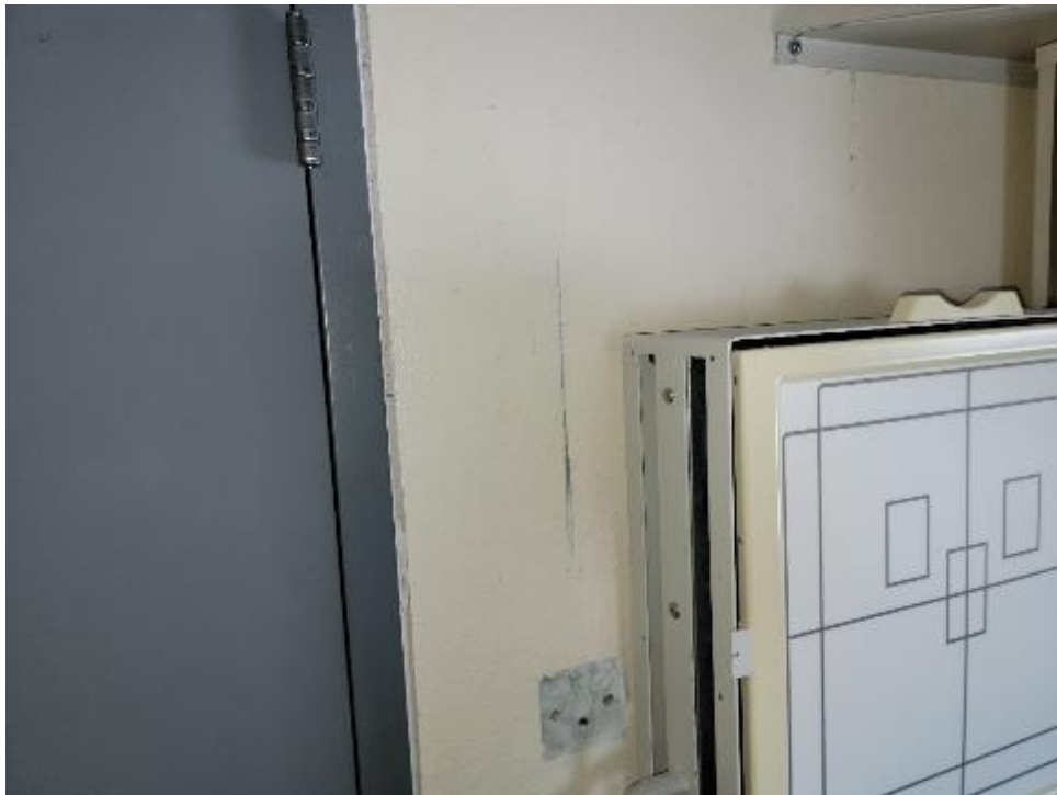
View of off-white paint on the walls (1.2 mg/cm 2 )
