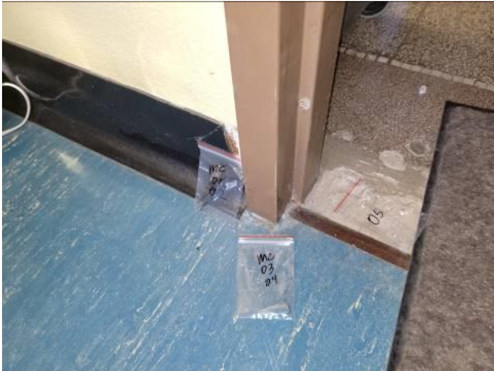
View of Blue Laminate Flooring (3% Chrysotile)
