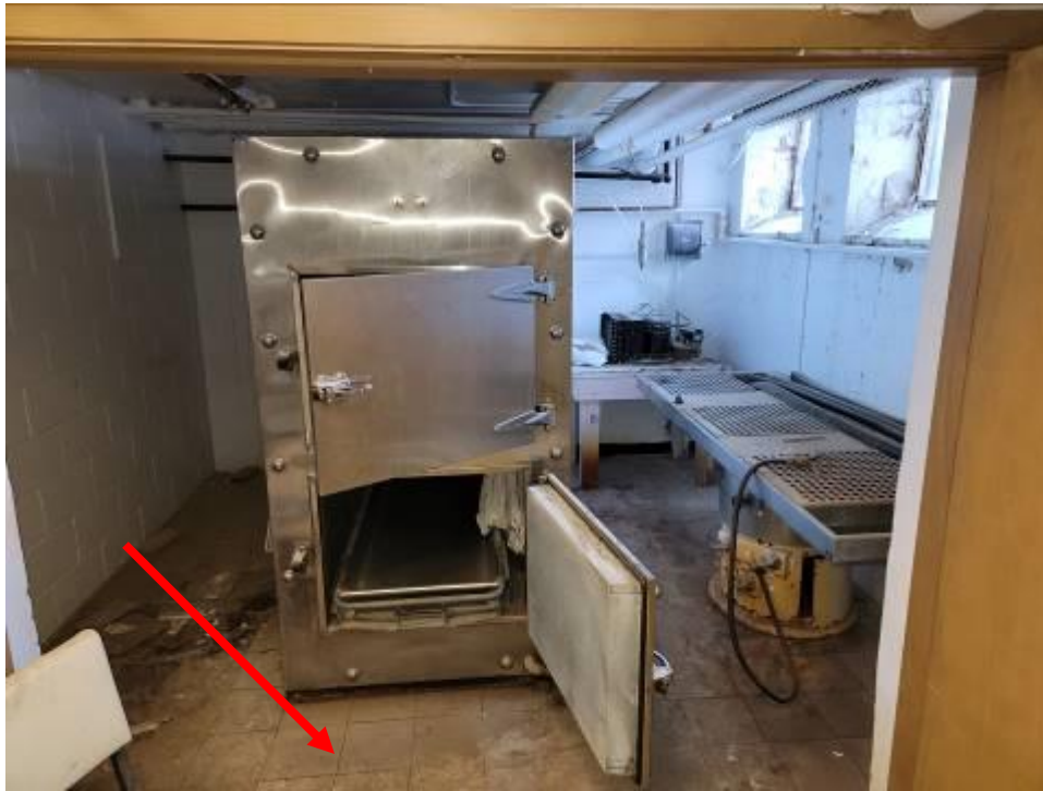
View of 9" x 9" Brown and gray/beige with pink, white, blue, brown VFT (3-5% Chrysotile)
