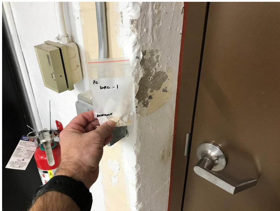
View of white paint on walls in basement. (0.048% wt)
