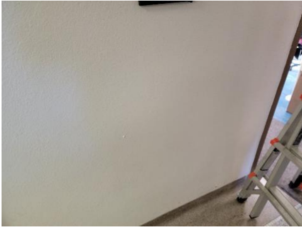
View of gray paint on plaster walls. (0.8 mg/cm 2 )
