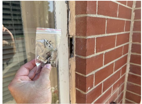
Photo #2 Looking at the exterior window caulking. (DIS-3, 20-35% Chrysotile)
