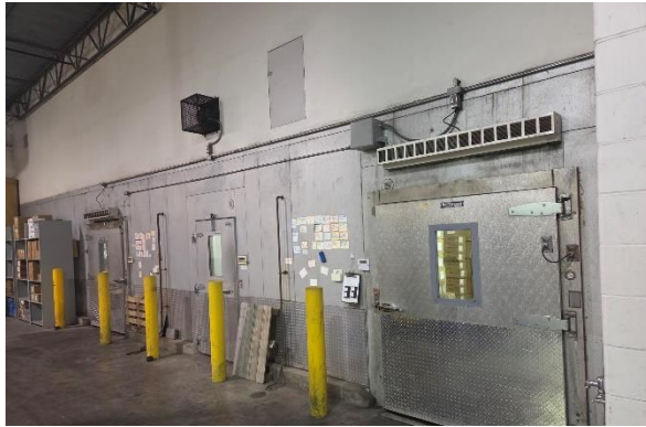
Photo #1 Warehouse W. Overview of South Freezers (no ACM or Pb paint)
