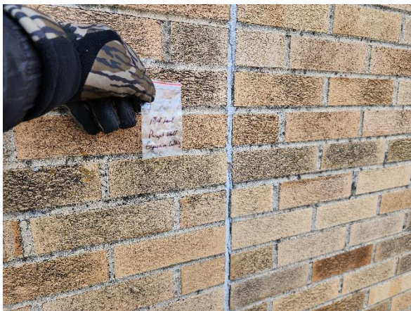
Photo #5 Sample #7. Asbestos containing expansion caulking on mid-level roof wall.
