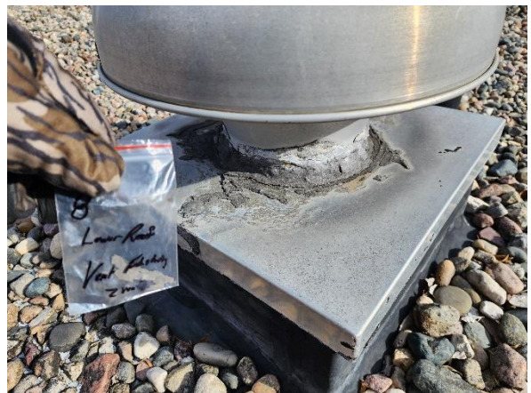
Photo #6 Sample #8. Asbestos containing vent flashing on lower roof.
