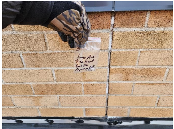
Photo #4 Sample #5. Asbestos containing expansion caulking on lower roof parapet
