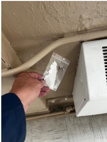
Photo #9 Paint Sample PC-4 – Plaster wall in Room ED3-12.
