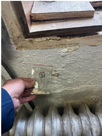
Photo #3 Sample #5 – Wall texture. Room ED3-18.
