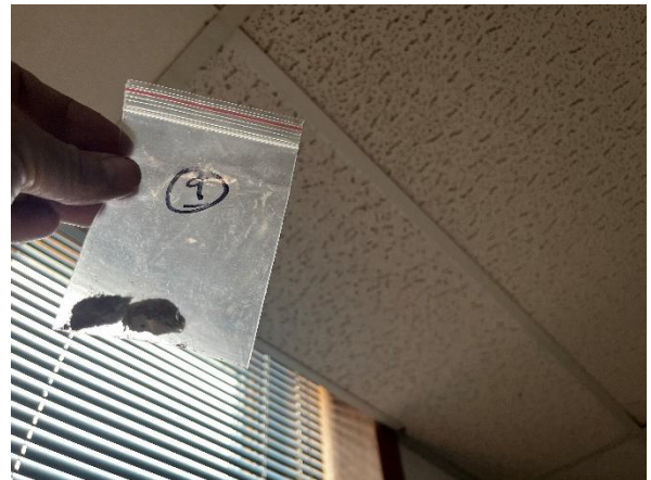
Photo #10 Sample #9 – 2'x4' Ceiling Tile in Room ED3-24.
