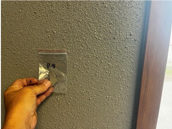
Photo #13 Paint Sample PC-5. Plaster wall in Room ED2-16
