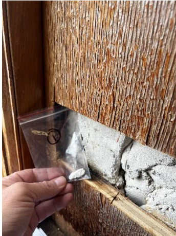
Photo #1 Sample #1 – Concrete outer wall. At NW Window in Room ED3-18.
