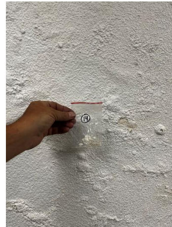
Photo #16 Sample #14 – Wall texture in Room ED1-12.
