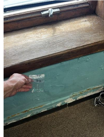
Photo #14 Paint Sample PC-6. Plaster Wall in Room ED2-17.
