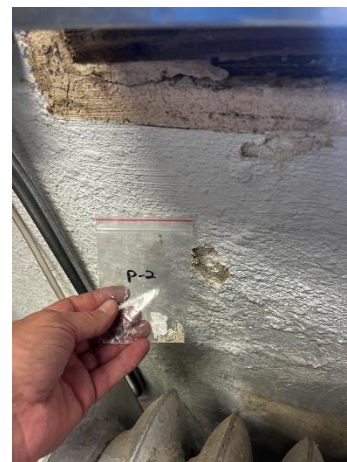
Photo #6 Paint Sample PC-2. Wall below NW window in Room ED3-18.
