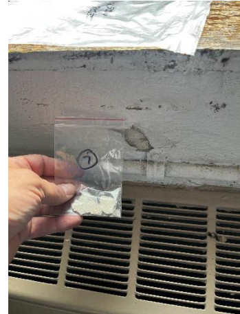
Photo #8 Sample #7 – Plaster wall in Room ED3-14.
