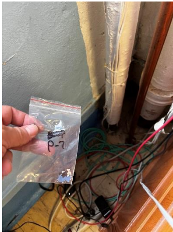
Photo #15 Paint Sample PC-7. Plaster Wall in Room ED2-26.
