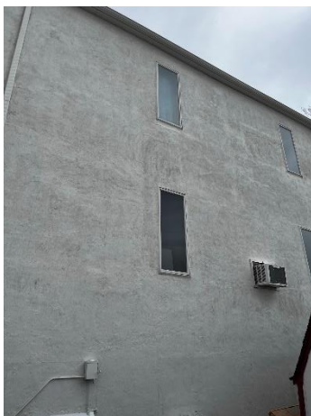
Photo #17 View of Building Exterior.
