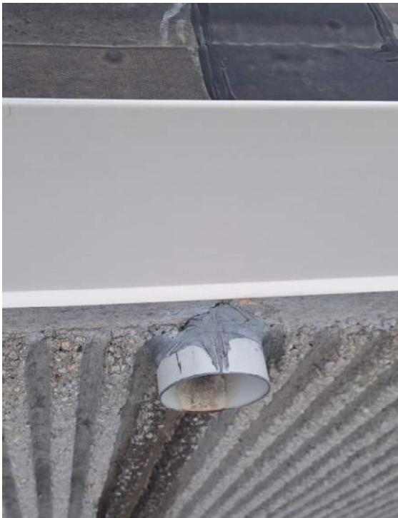
BUILDING EXTERIOR - OVERFLOW PIPE SCUPPER
