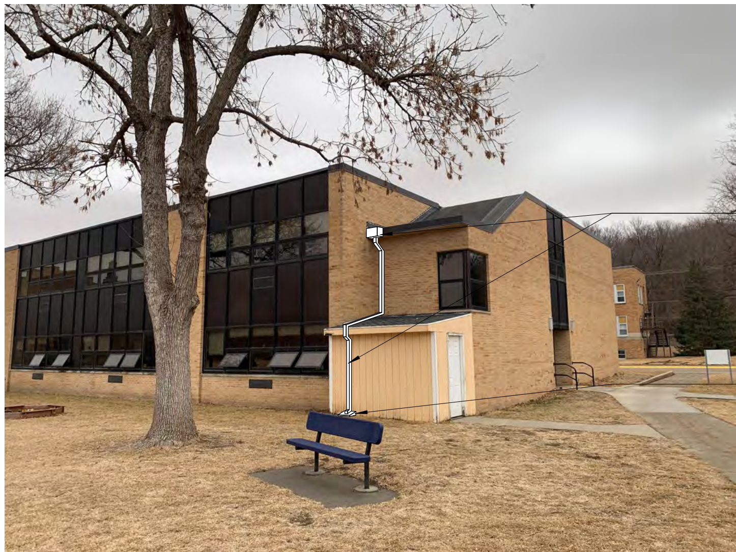
2 NEW SCUPPER AND DOWNSPOUT
