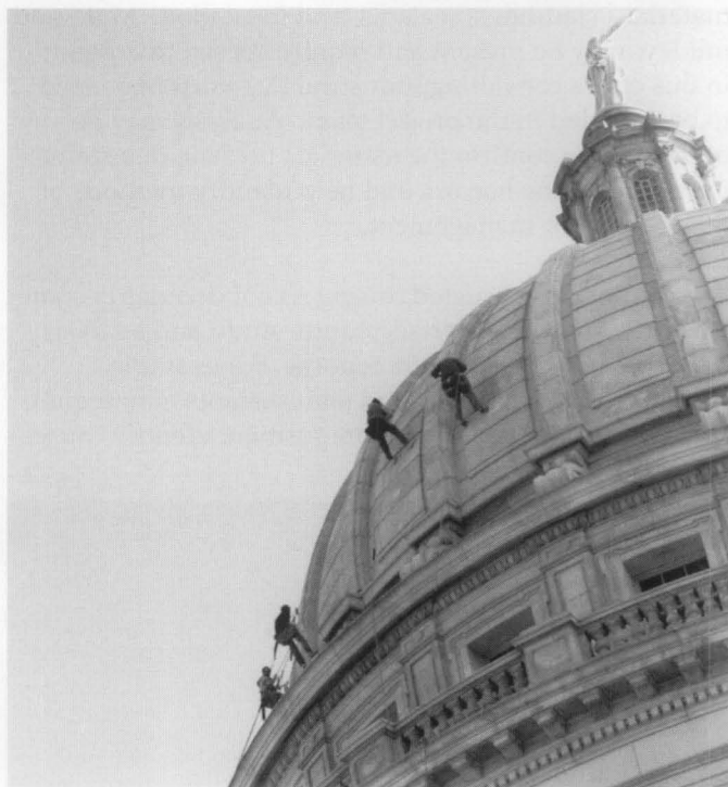
Figure 11. The use of special access methods may be necessary for close-up investigation of building elements. At the Wisconsin State Capitol, project architects and engineers used rappelling techniques. Photo: Wiss, Janney, Elstner Associates, Inc.
