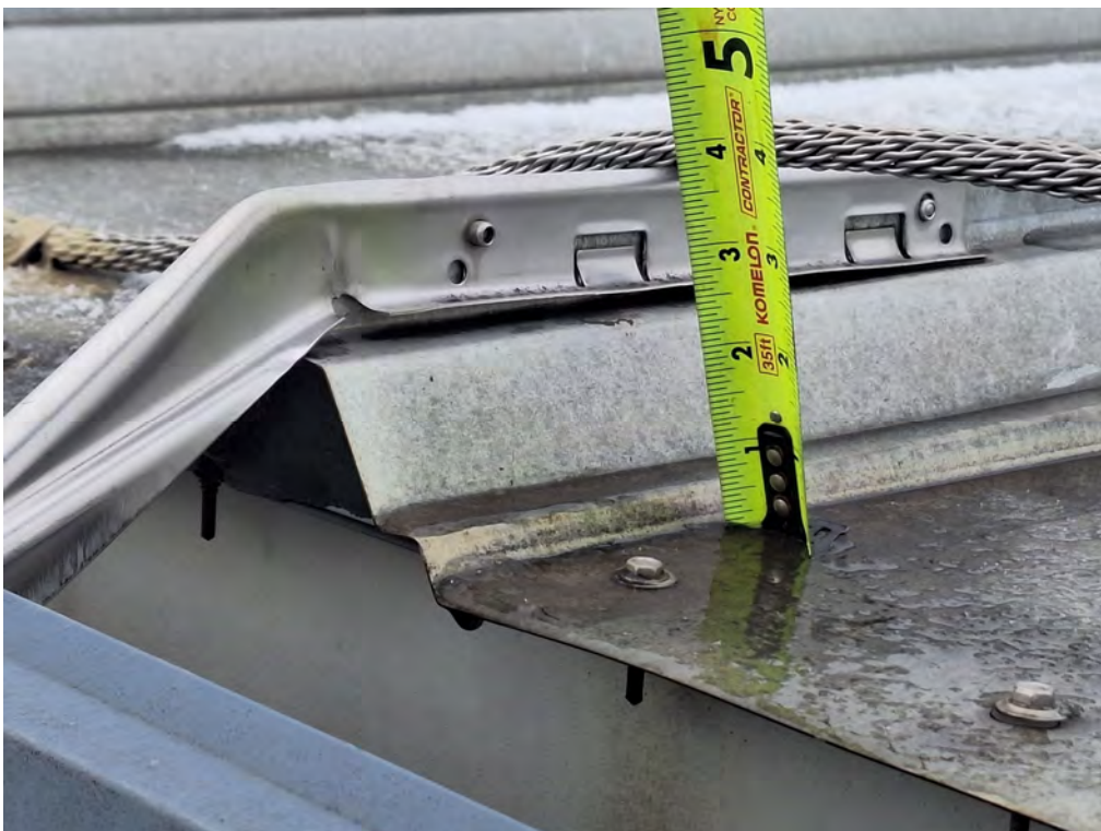
TYPICAL TRUNCATED SEAM AT GUTTER
