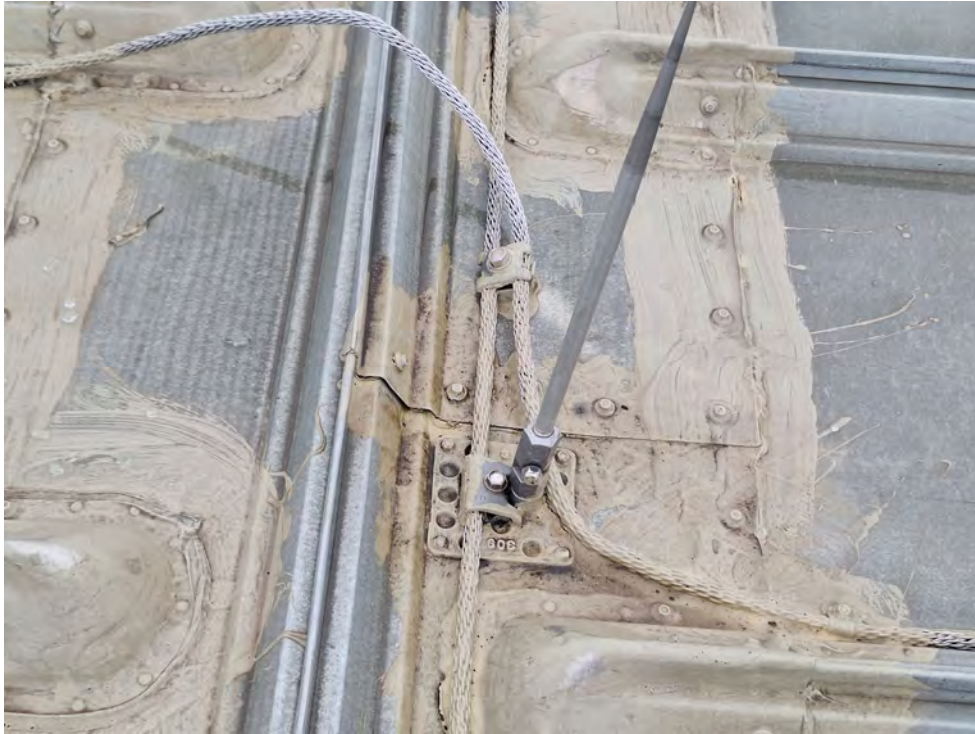
LIGHTNING ROD AND BASE CLIP
