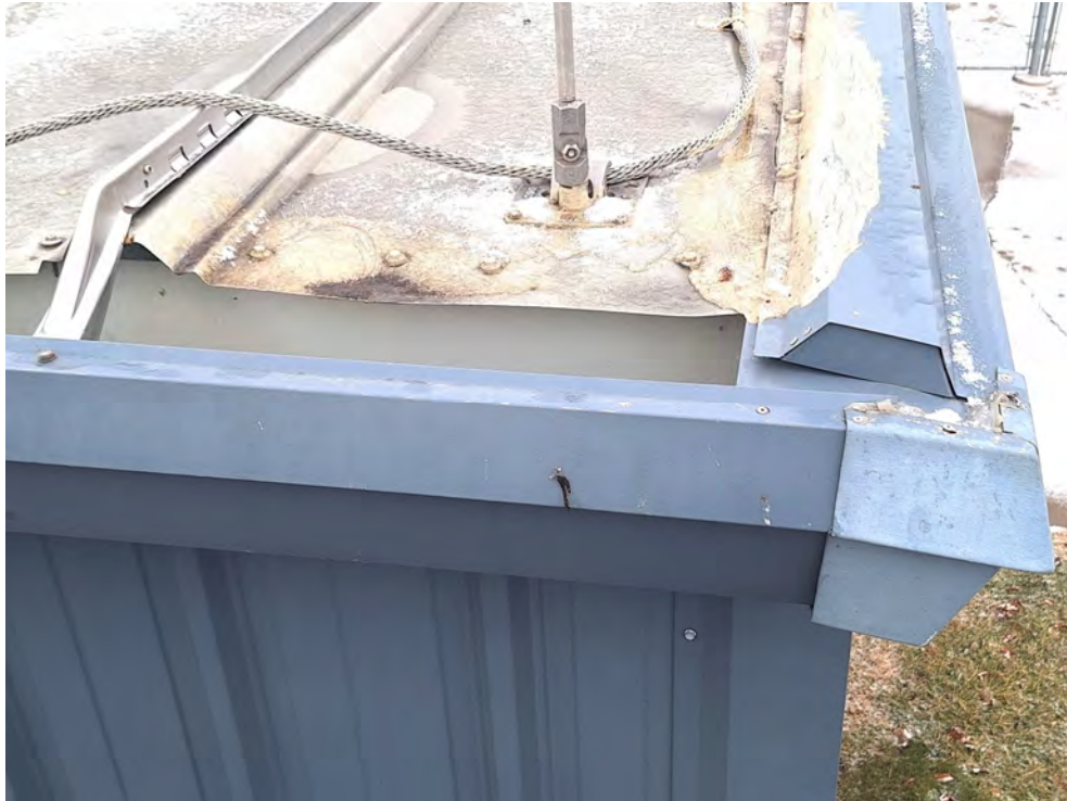
EXISTING GUTTER AND RAKE ENLOSURE AT CORNER
