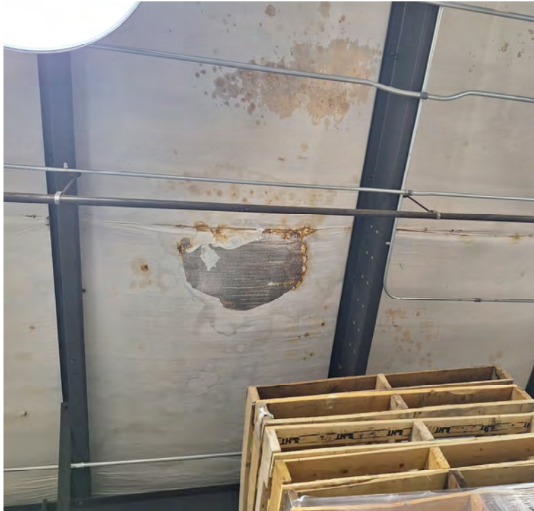
INTERIOR INSULATION PATCH AREA AT EAST LOADING DOCK
