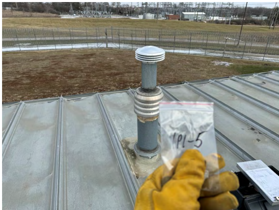
Example of caulking/sealant on vent stacks that were inspected and sampled.
