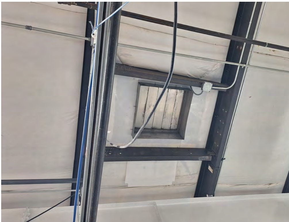
INTERIOR INSULATION PATCH AT EXHAUST FAN TO BE REMOVED
