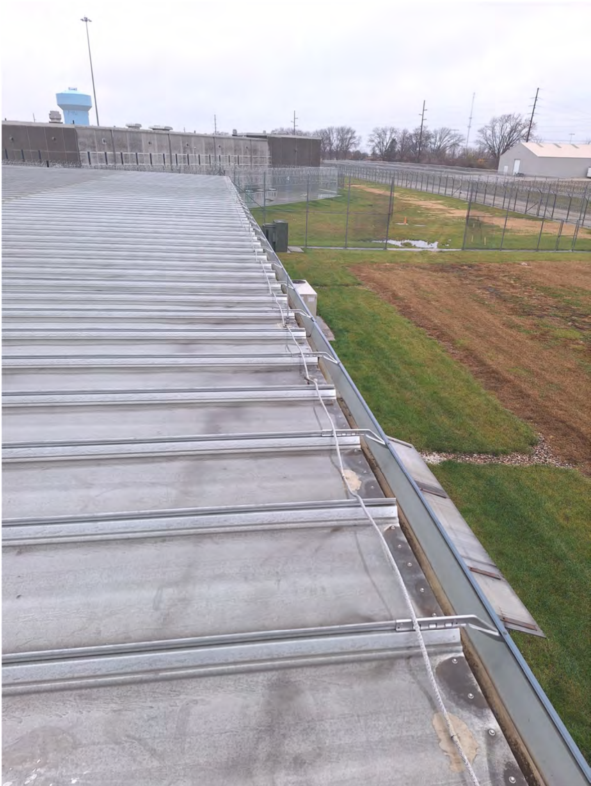
EXISTING GUTTER AND LIGHTNING CABLE
