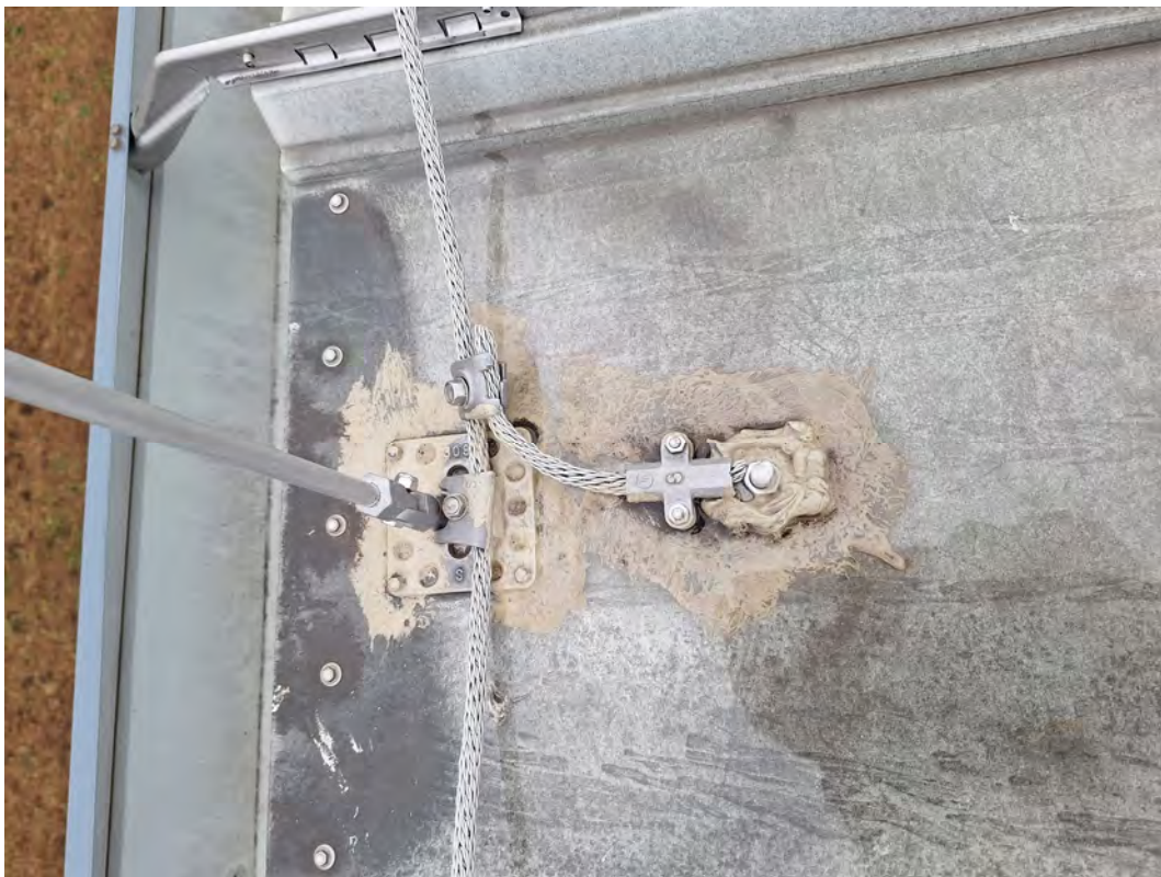
LIGHTNING ROD AND LIGHTNING CABLE PENETRATION
