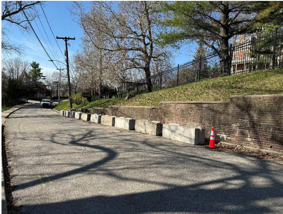
View of the retaining wall, looking southwest.
