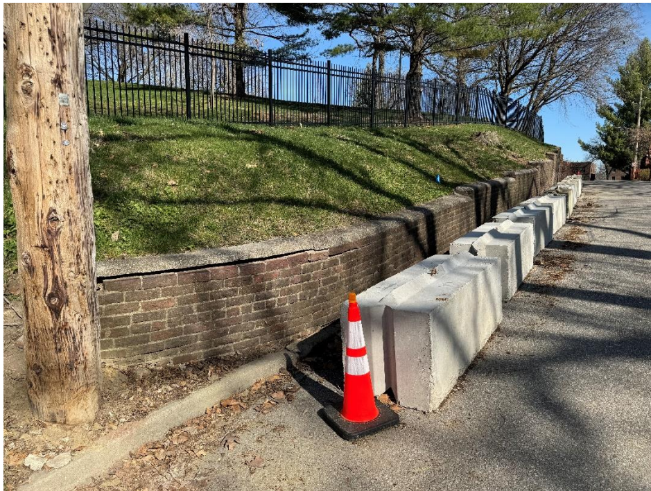
View of the brick retaining wall, looking north.
